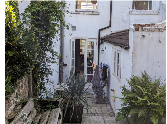
06. Existing rear of the property
