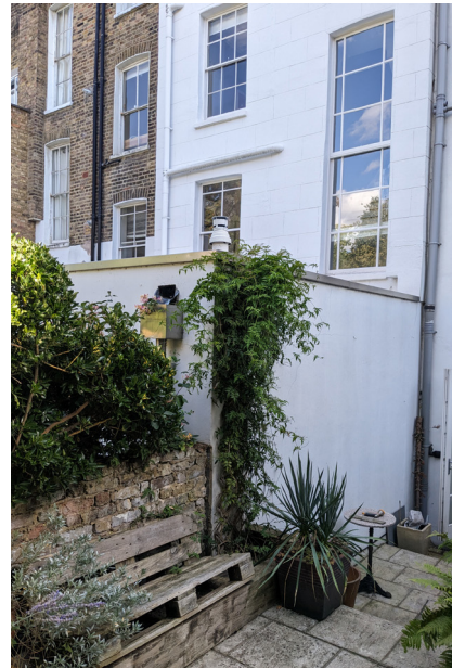
05. Existing rear of the property
