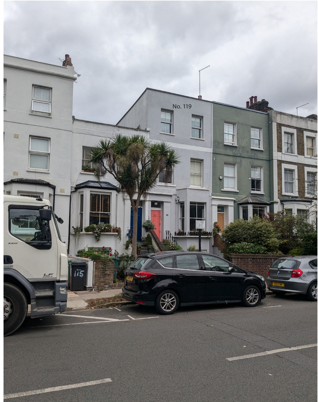
12. Photo of 117, 119 & 121 stepping back from the building line
