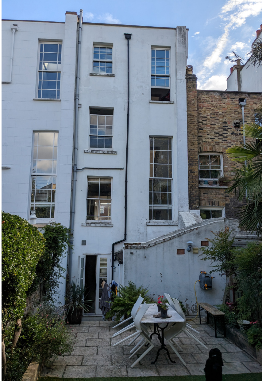
04. Existing rear of the property
