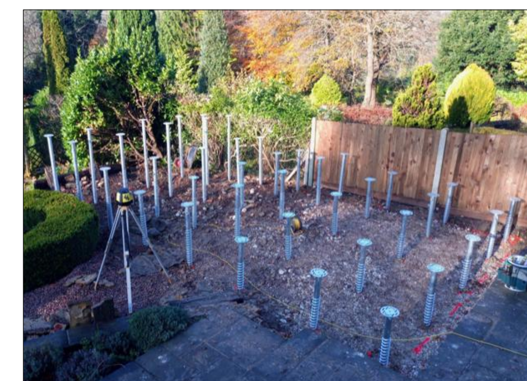
Ground Screws During Typical Installation
