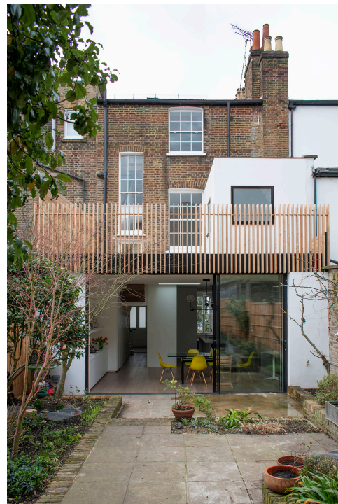
Fig.03 (above) The previous rear elevation and current rear elevation of no.108 Torriano Avenue. The new proposals sensitively retain the existing balustrade and general scale and massing of the existing elevation. The previous rear elevation had a wider closet wing that sat partially over the existing sash window at first floor level.
