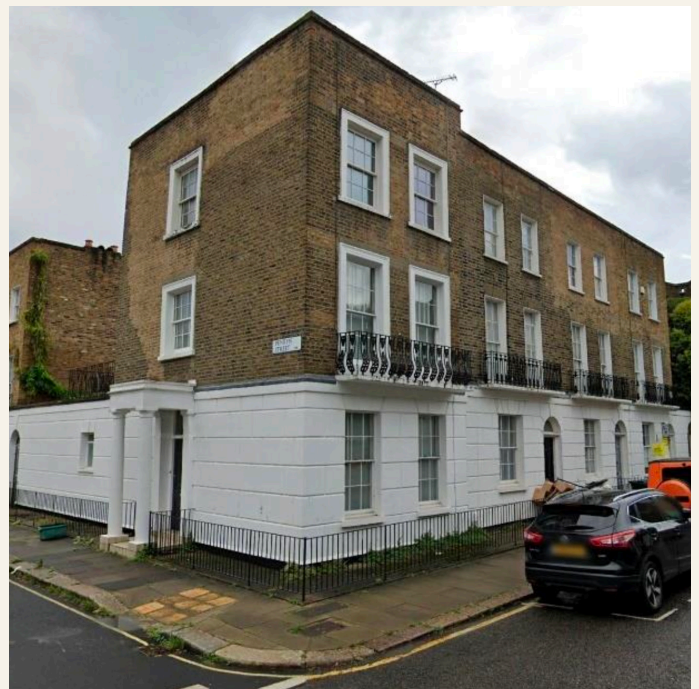
Fig. 1: External view of the property
