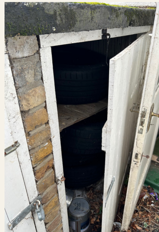
Fig.3: Photo of existing external store
