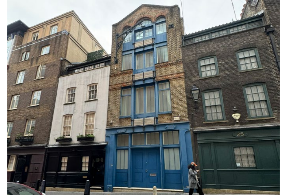
View 4: Front View of 23 Mercer Street nestled between number 21 and 25.
