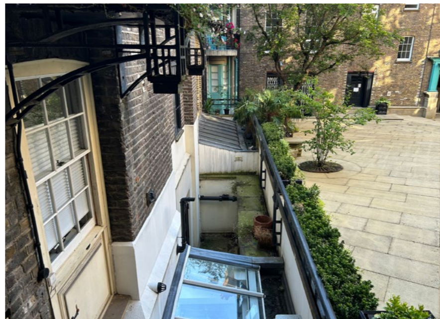
View 7: Rear lightwells to Mercer Street showing a combination of glazed infills and open lightwells
