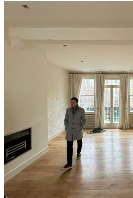
Existing Timber beam at 1st floor with chimney addition concealing strut
