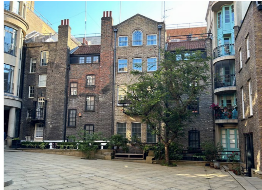
View 5: View of the rear of 23 Mercer Street from Ching Court
