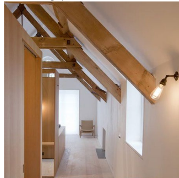
Joinery to underside of beams
