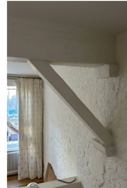
Original strut location between white painted brick and timber beam
