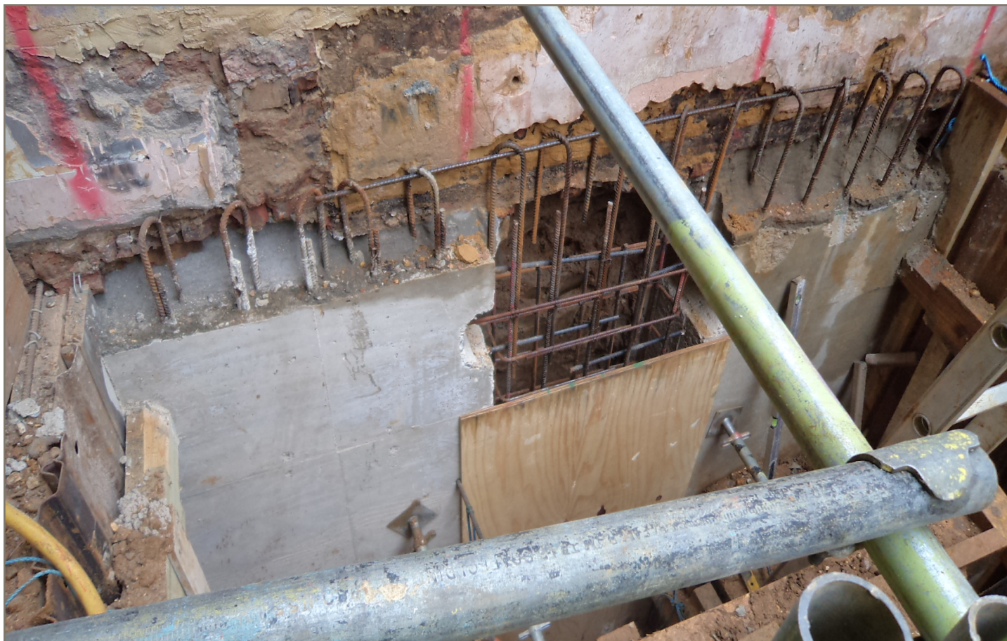
Example of retaining wall construction in a 'hit and miss' sequence
