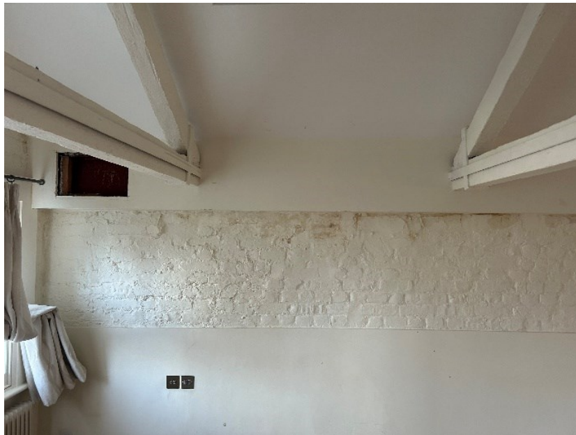
Figure 21: The steel positioned on the party wall with no.25 Mercer Street, with the roof trusses bearing onto it.
