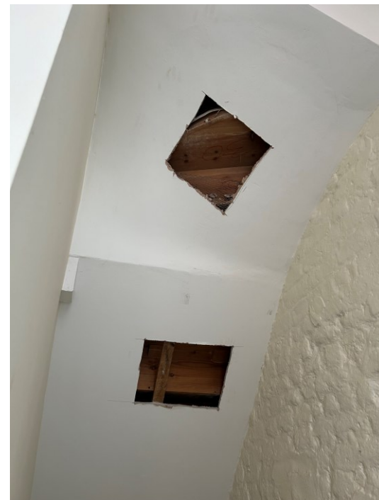
Figures 18 & 19: Plans from 1985 show the approved layout of no.23 Mercer Street including the staircase, which his clearly annotated as “new softwood stair” (left) and limited opening up works to the soffit of the staircase confirm that this is constructed of modern timber with a modern metal mesh and gypsum plaster finish (right).
