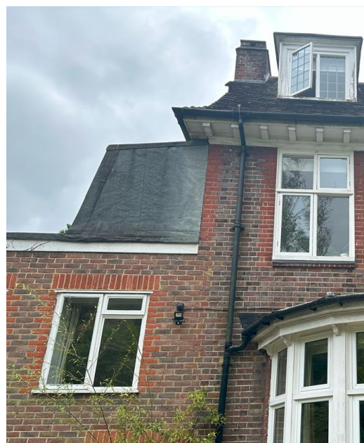
Figure 7: Photograph of intersection between main building and side projection
