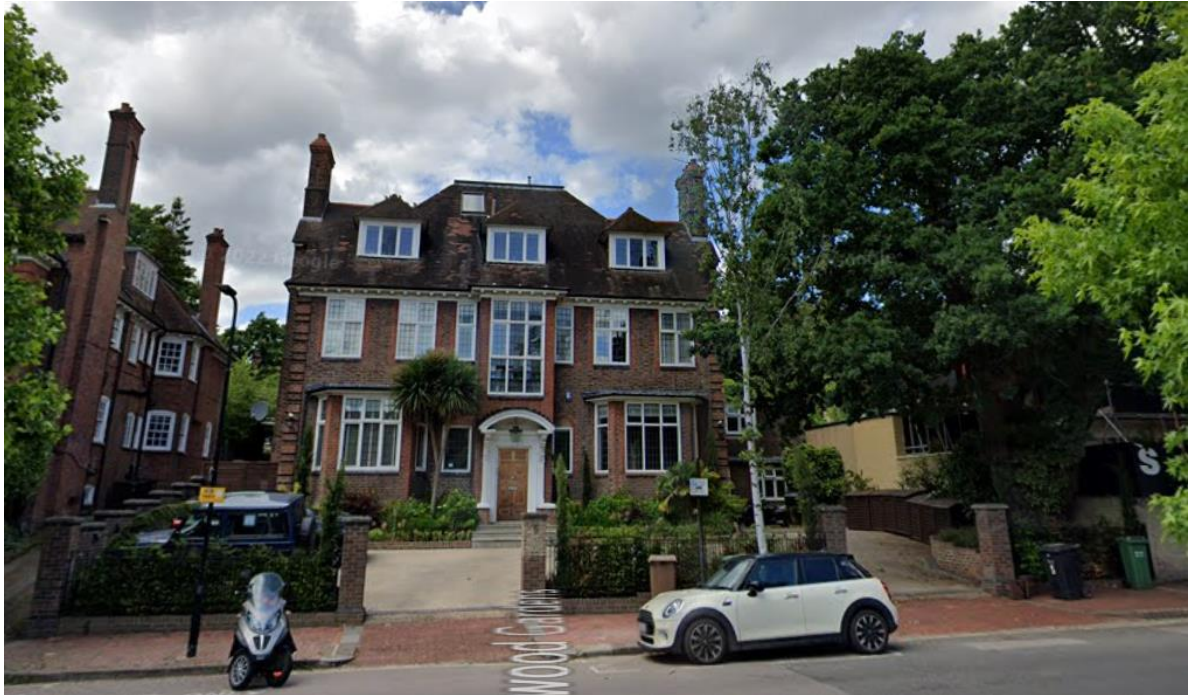
Figure 3: Google Streetview imagery of front elevation of the application property (June 2022)
