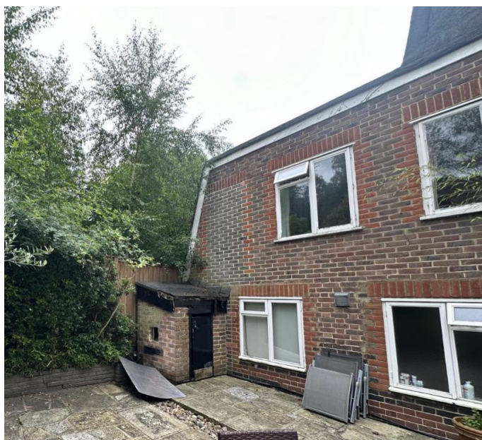
Figure 6: Photograph of existing projection's rear elevation
