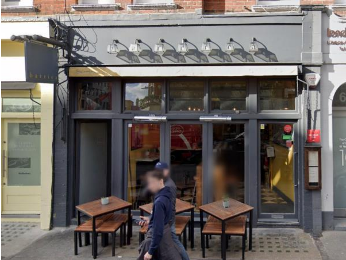
Heaters on Barrica Restaurant
