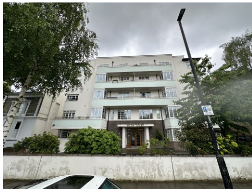
Figure 2: The front façade of Hylde Court.
