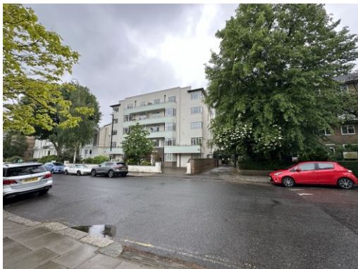
Figure 12: A close range view of the front façade from St Albans Road.
