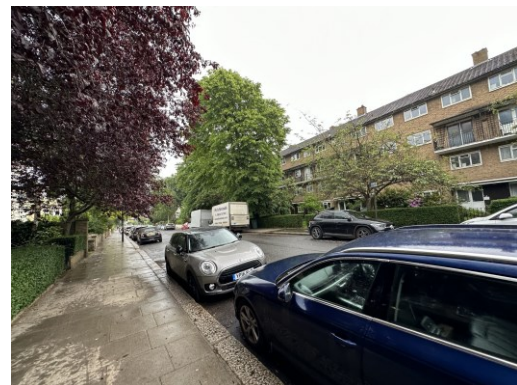
Figure 14: A view looking west along St Albans Road towards the site, with the tree in the forecourt of the site obscuring views of the building.
