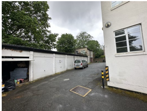
Figure 10: The garages at the rear of the site and the tarmac area between them and the rear of Hylda Court.
