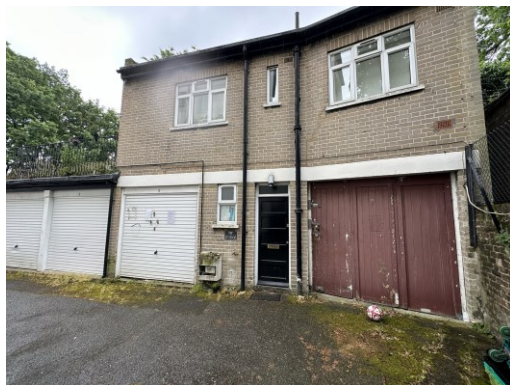
Figure 11: The two storey caretaker's cottage in the SW corner of the site.
