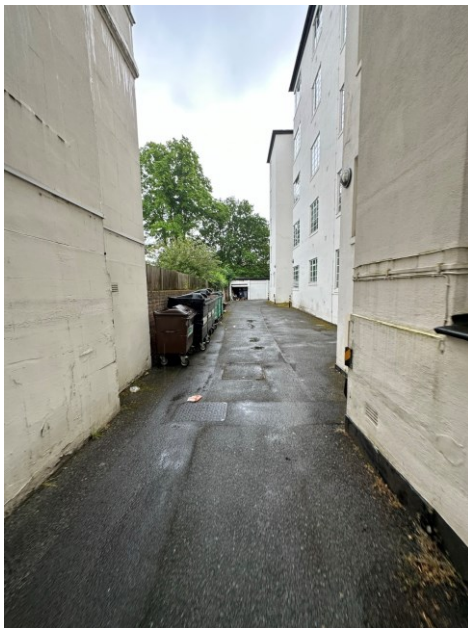
Figure 16: The tarmac covered driveway to the east of Hylda Court.
