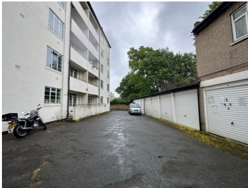
Figure 15: The existing area to the rear of Hylda Court, with the garages and caretaker's house on the right.
