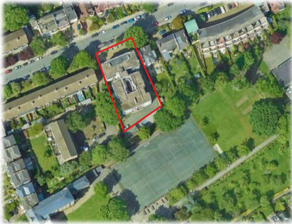
Figure 1: Aerial Image of the site with an approximate red line boundary (Google Maps)
