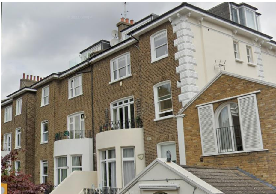
No's 21 & 22 Belsize Square
