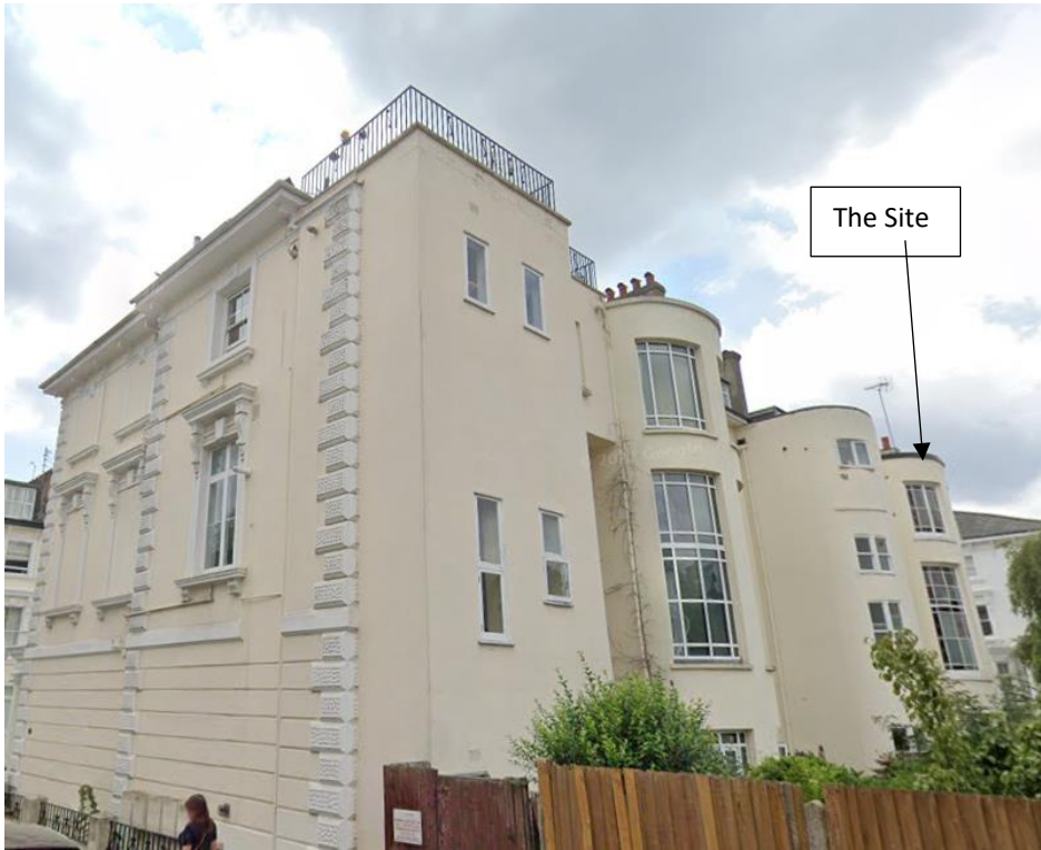
No's 27-30 Belsize Square
