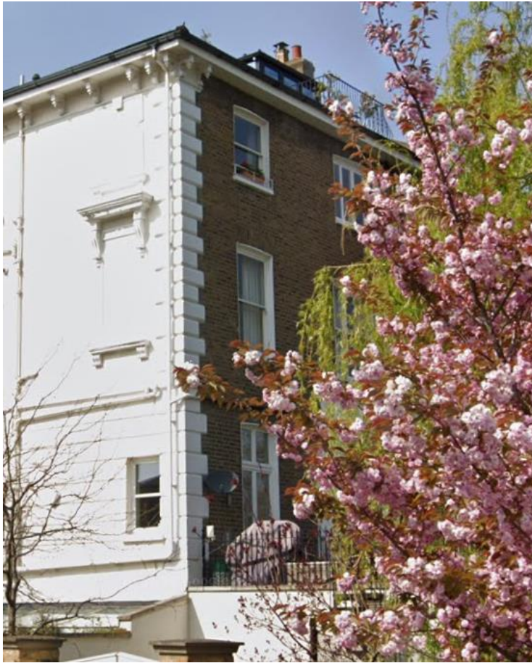
No.1 Belsize Park roof terrace (approval ref: 2010/3073/P)
