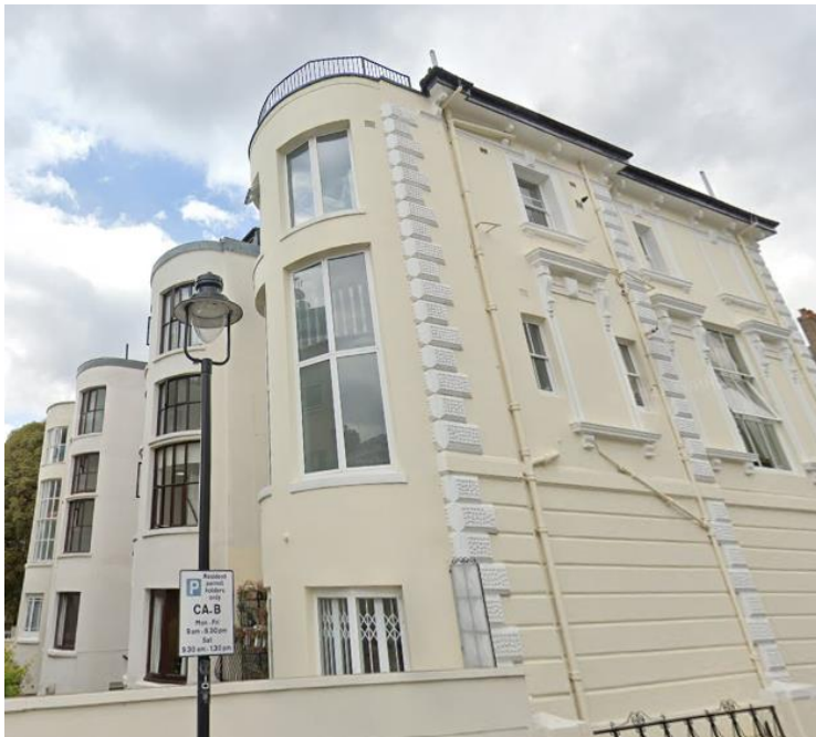
No's 23-26 Belsize Square
