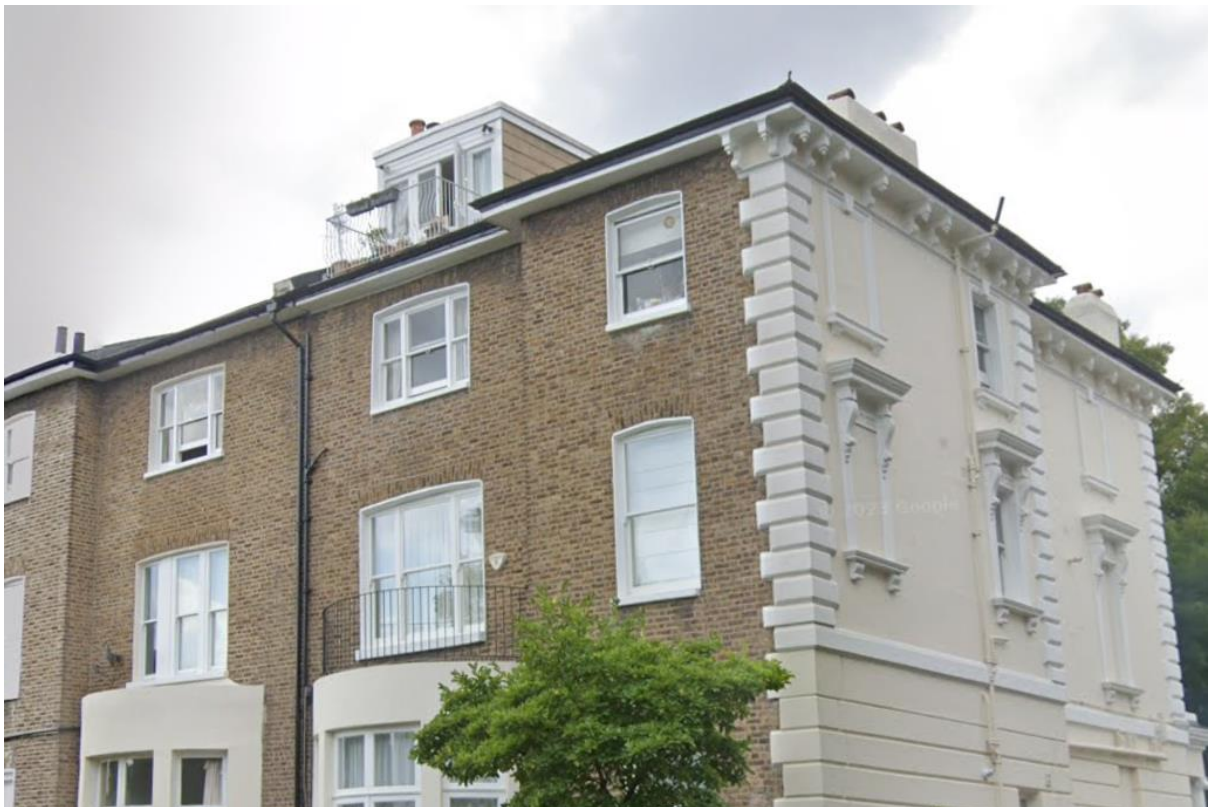
No.8 Belsize Park roof terrace (approval ref: 2007/3011/P)
