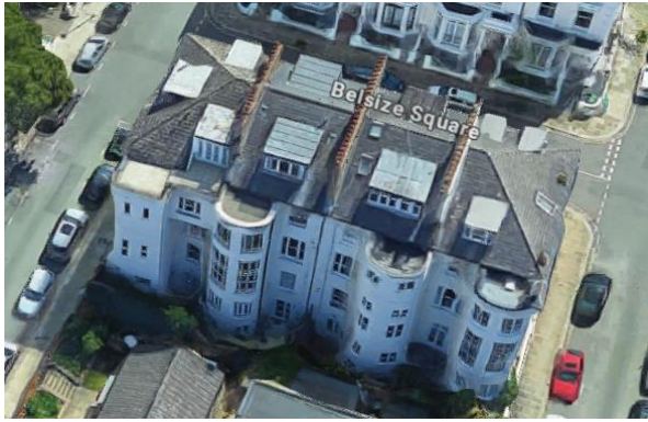
Rear elevations of No.'s 27-30 Belsize Square
