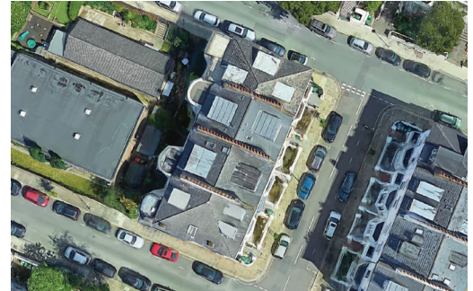
Aerial view of the application site
