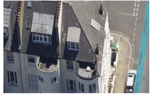
Aerial view of the application site
