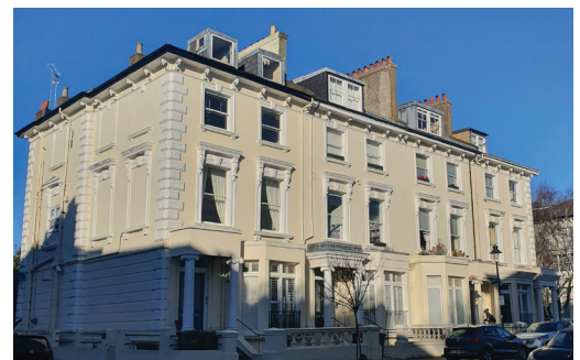
Street view of No's 27 - 30 - showing dormer overlapping hip line/construction
