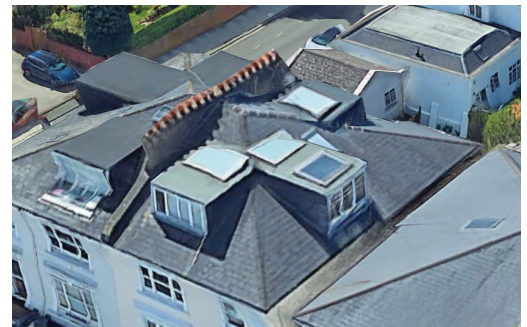
2006/3108/P - As built dormers to No.21
