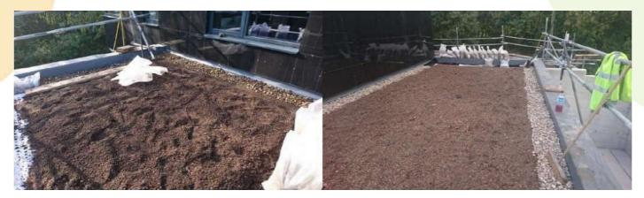
The roof area should be dipped to ensure the substrate depth is as required. The specified substrate depth must be achieved with an additional 10% settlement factor allowed for.
