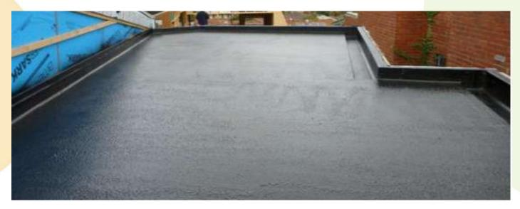
Ensure the roof is complete and watertight. Check that roof is a safe working environment i.e. edge protection/scaffold or man safe system is in place. Have lifting equipment ready to lift materials to the roof. Ensure all other trades have finished working on roof before starting. Double check with site that the roof has been leak tested prior to our works and notify the contracts manager immediately if you spot any potential leaks.
