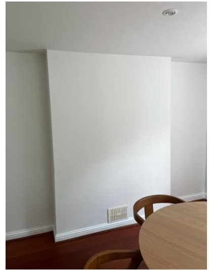
Figures 22 and 23: Lower ground floor kitchen (left) without a chimney breast and rear lower ground floor room with bare chimney breast (right)
