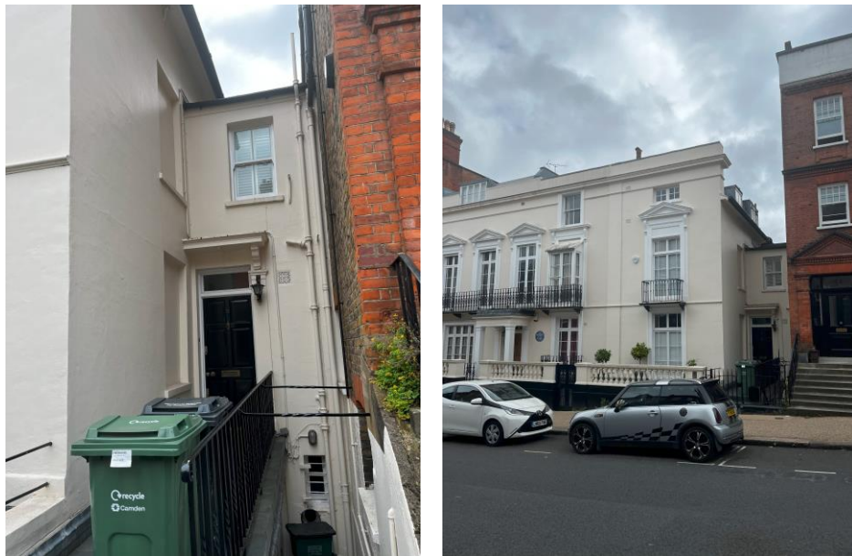
Figures 8 and 9: Former front elevation of no.51, now the side elevation, with surviving earlier window openings present
