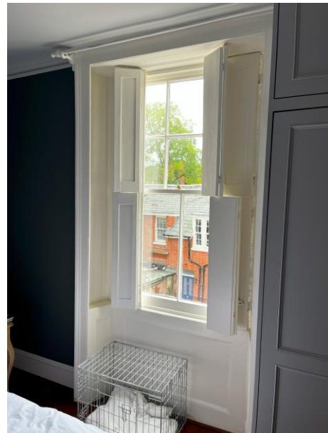
Figures 14 and 15: Photographs showing the window boxes and shutters present to the first floor rear room
