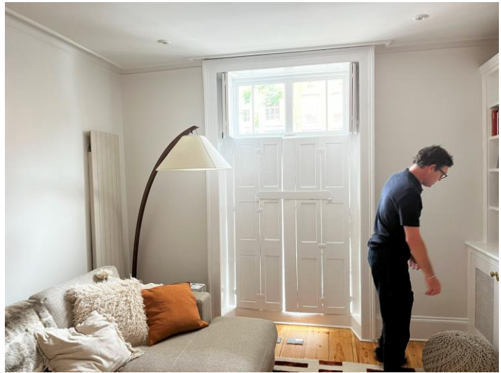
Figures 12 and 13: Photographs showing the decorative cornice and window architrave/shutters present to the ground floor front room
