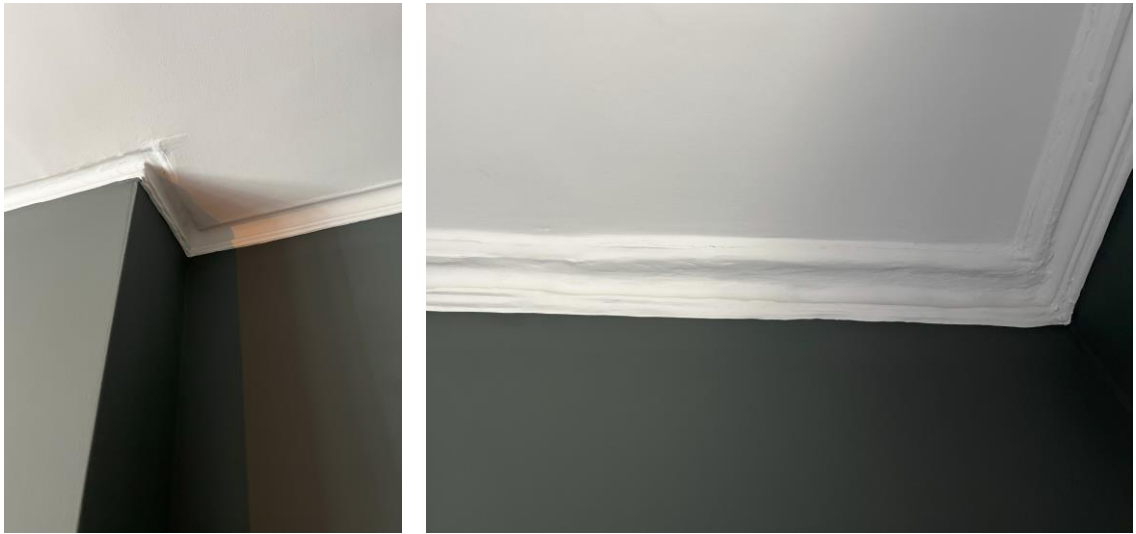
Figures 20 and 21: Photographs of the cornices present to the first floor front and rear rooms showing damage occurred through the over boarding of ceilings and poor quality repairs
