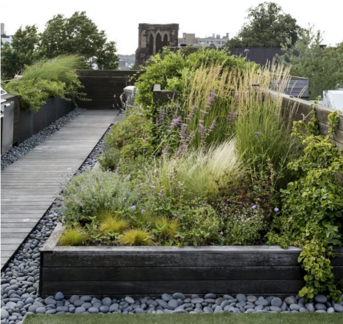
Photo 2: Proposed Construction : 200mm high timber-sided beds containing Bauder Intensive Landscape System, edged in stone pebbles.
