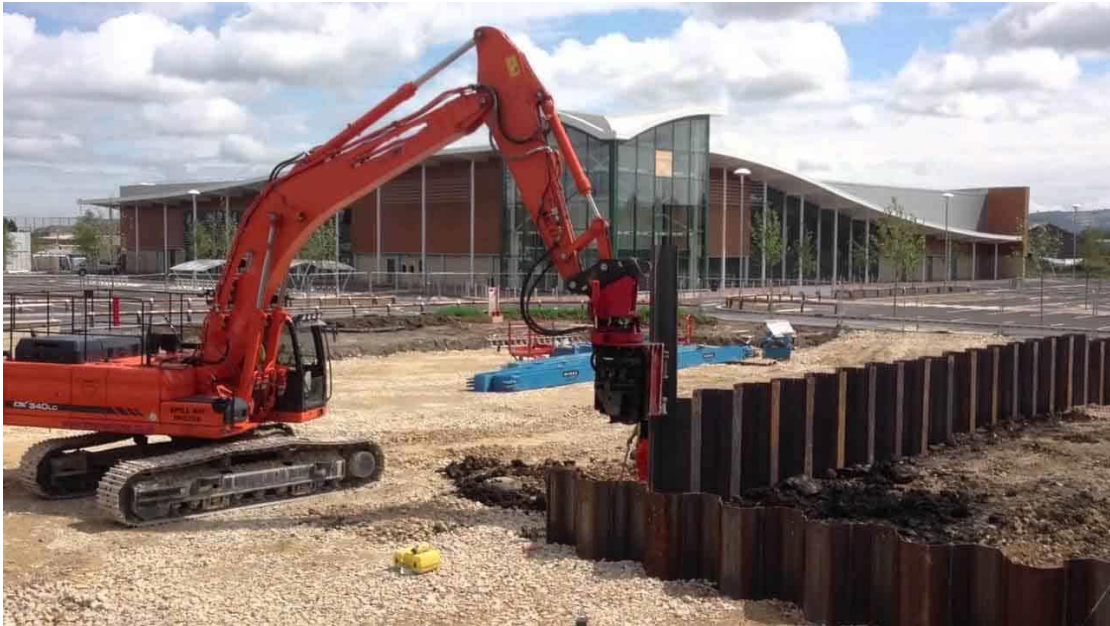
Insert D – Example of sheet pile excavation support
