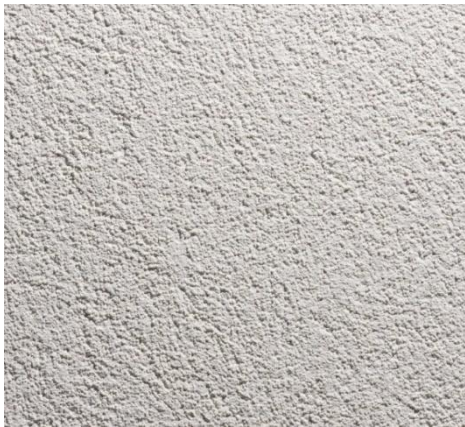
Figure 12 above _white render on main extension wall finish.
