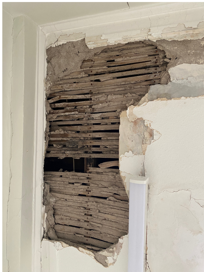
Lath and Plaster Ceiling
