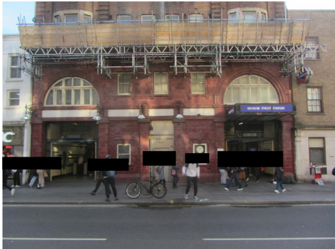
Front elevation: showing faience/terracotta facade of tube station
