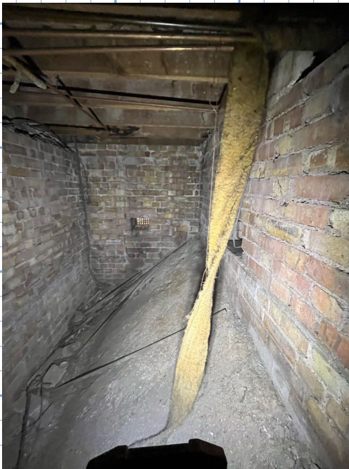
View North - behind existing corridor wall
