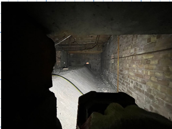
View South - beyond existing corridor wall
