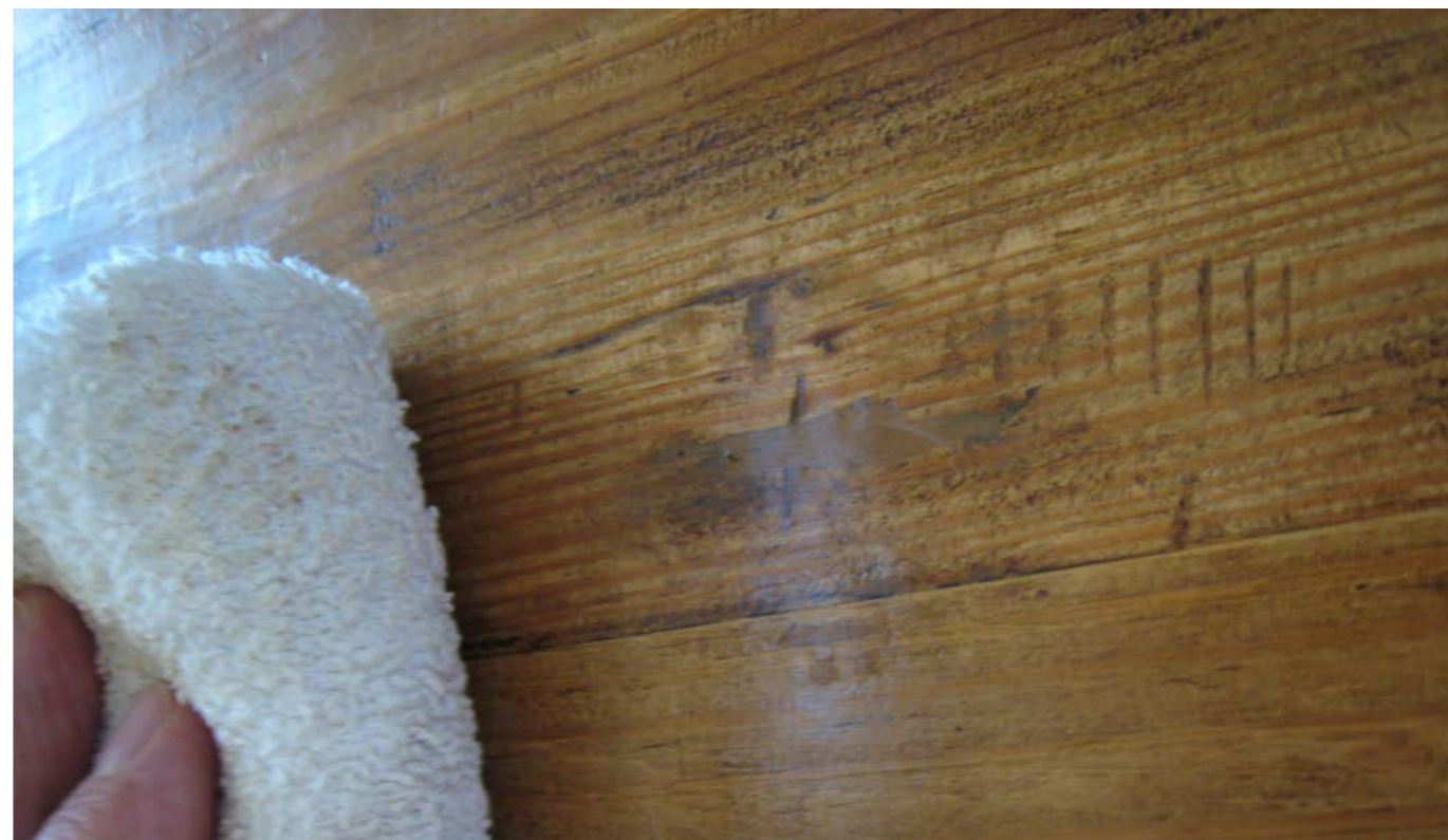
Surface polished/finished to match existing timber
