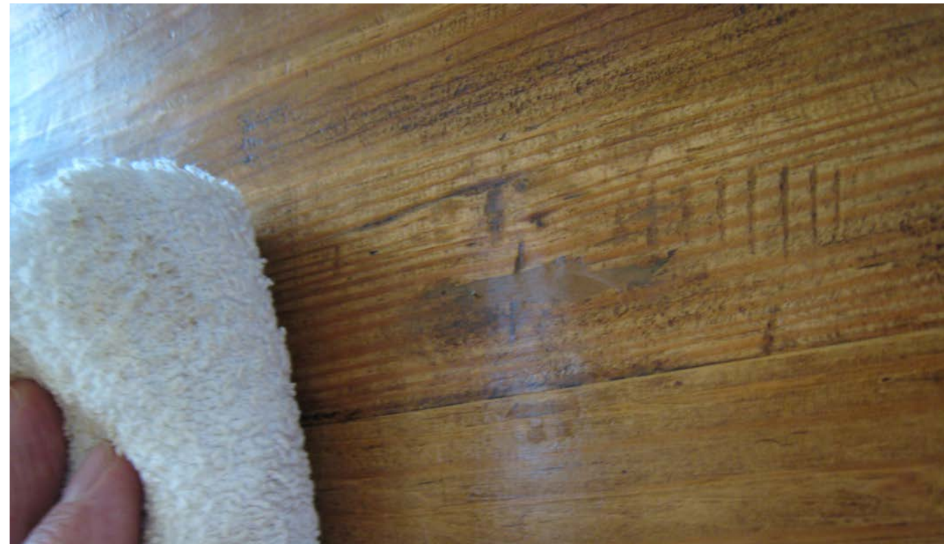
Surface polished/finished to match existing timber
