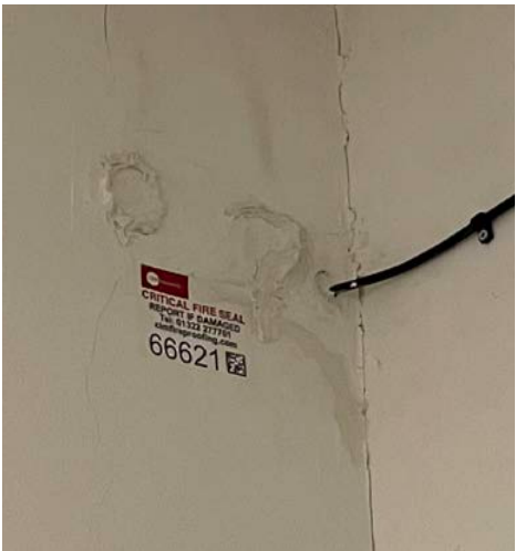
Existing service penetration
