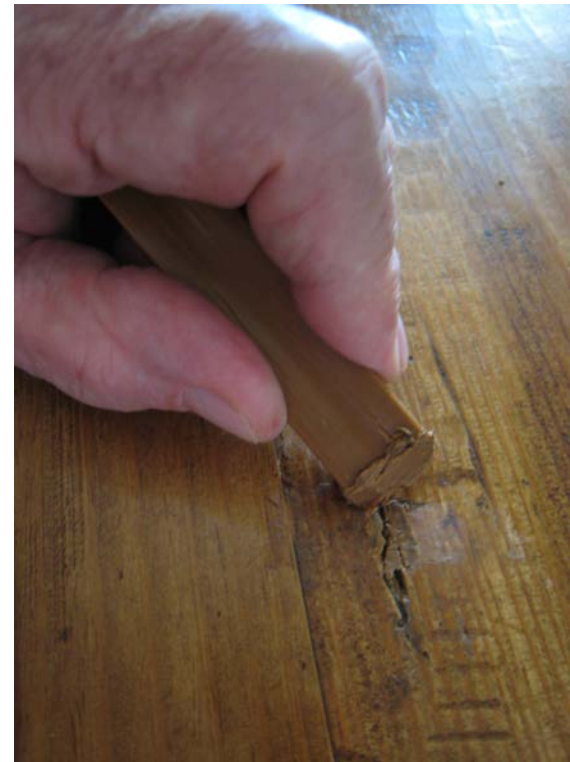
Minor wear filled with wax
