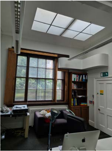
Above: Photograph of the existing window and mechanical vent. Shown to the right: Drawings detailing S.Glazing Type D2, showing vent boxing throughout room A/2/007
