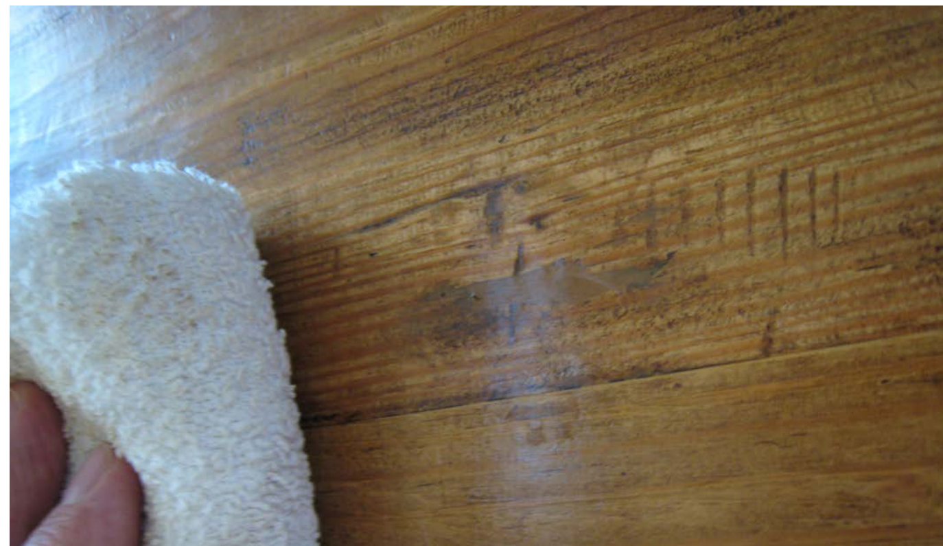
Surface polished/finished to match existing timber
