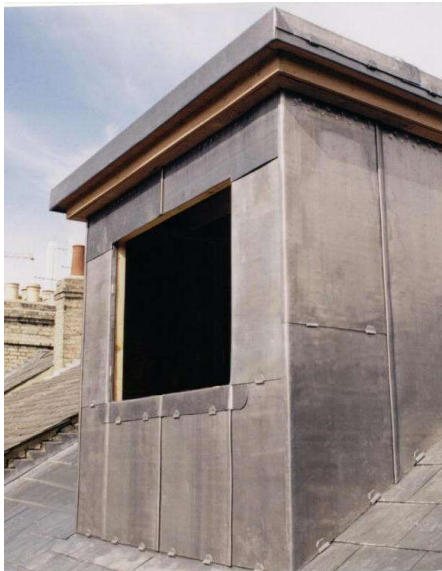
Image 06 - Lead clad dormers
