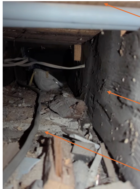
Photo taken between ceiling and floor boards (first to second floor)
