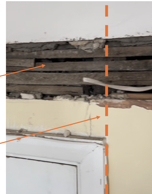
Photo taken of spine wall at first floor level
