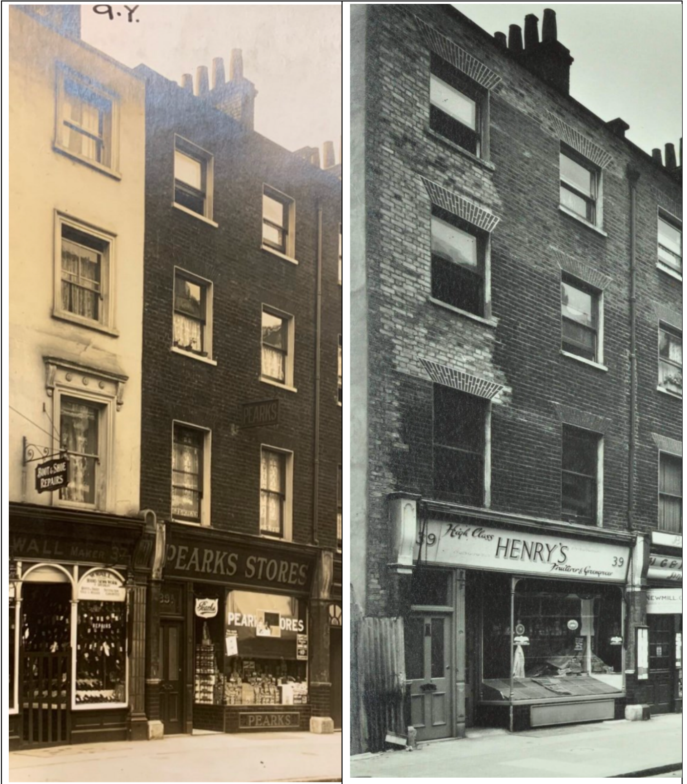
Figure 2: Credit Jon Lowe Heritage Report. Left: Picture of 39 Marchmont Street elevation dated 1930 (pre WWII) the adjacent building is still present and the façade brickwork is uniform. Right: Picture taken 1956, façade brickwork has been extensively replaced and the party wall has been rendered, the adjacent building has been demolished
