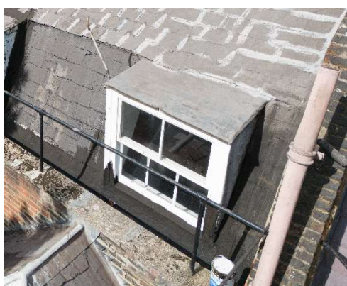
Lower sash of R3.2, assessed to be original fabric
