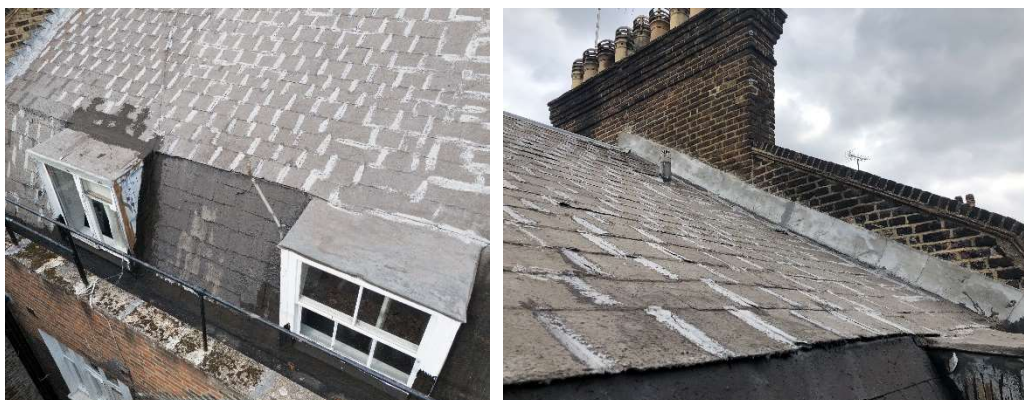
Main roof covering in very poor condition
