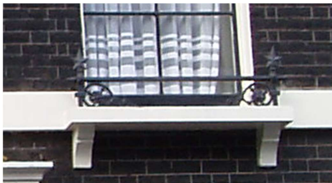
Style of bracket to be replicated (71 Gower St)
