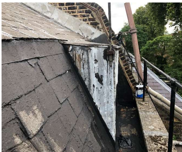
Existing steel parapet handrail to be removed
