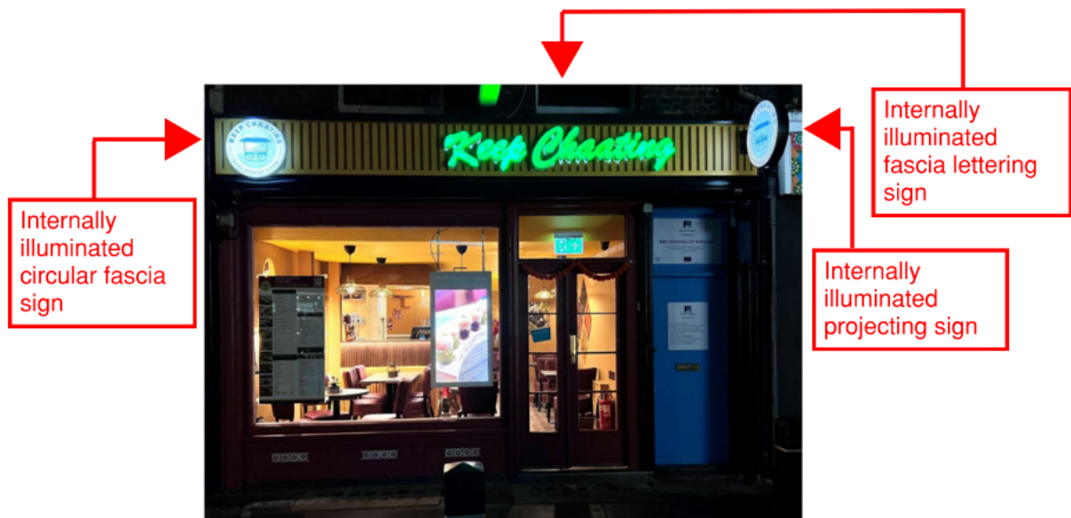
Image 2 – photograph of original proposals (front elevation of application site viewed at night)
