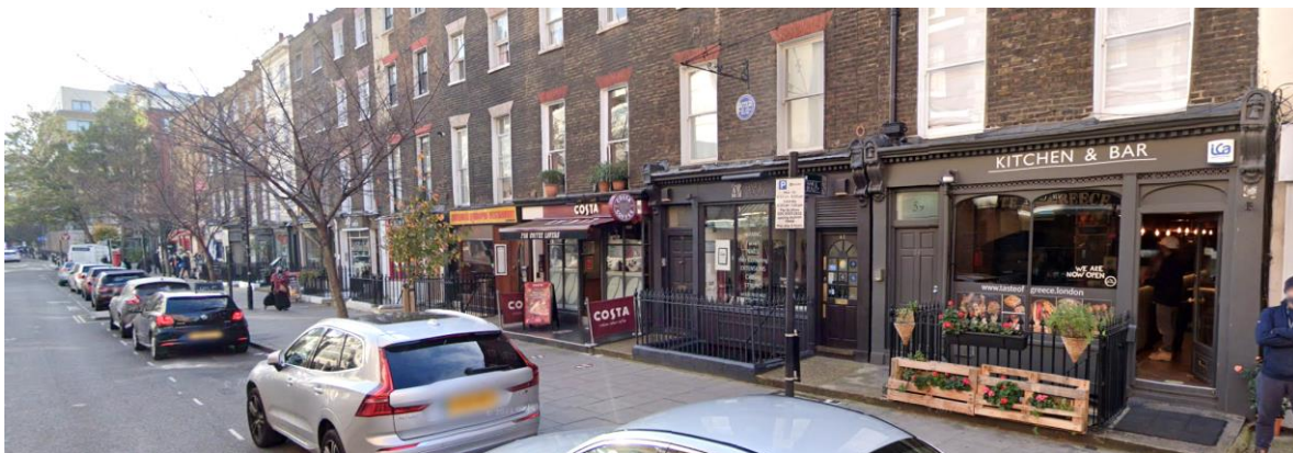
Figure 1. Existing front lightwells with stairs along the Marchmont Street frontage of the buildings in the Terrace with the Site visible on the far right (Google Streetview).
