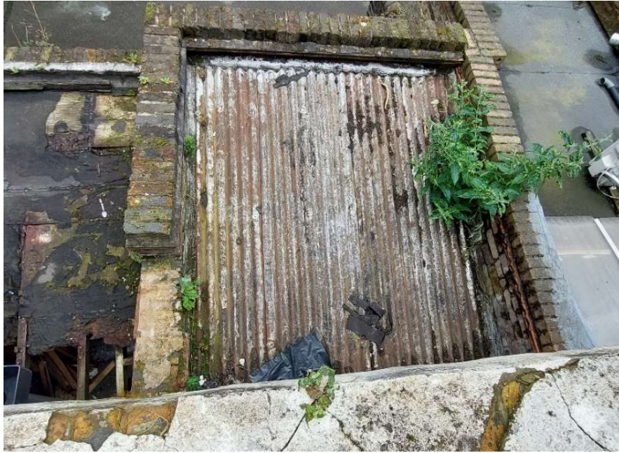
Image 21- Photograph of the roof over external store room which is proposed to be replaced with warm flat roof
