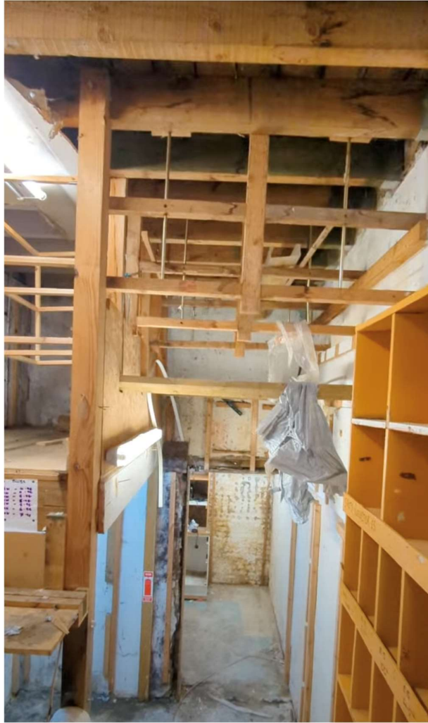
Image 16- Photograph of the 1 st floor rear roof terrace from inside shop and unoriginal timber mezzanine structure. It is proposed the roof is to be replaced with new warm roof and mezzanine structures to be removed.
