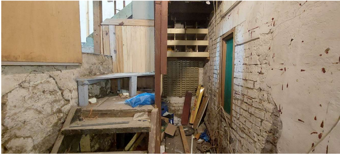
Image 12- Photograph of back of shop showing later addition timber stairs and the unoriginal window. Stairs and window are proposed to be removed. A new opening in the location of the removed window to be created to allow access.
