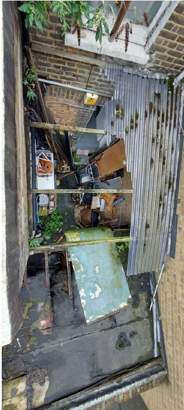
Image 20- Photograph of the failing roofs over the rear courtyard from above which are proposed to be removed
