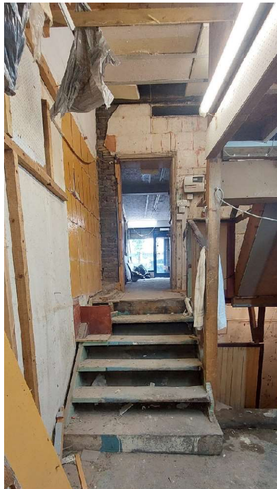
Image 13- Photograph of later addition unoriginal timber stairs and mezzanine floor at the back of shop that is proposed to be removed. Floor in this area is proposed to be levelled with front of shop.
