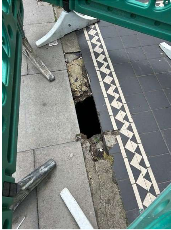
Image 10- Recent photograph of the failing lightwell infill at the front of the
