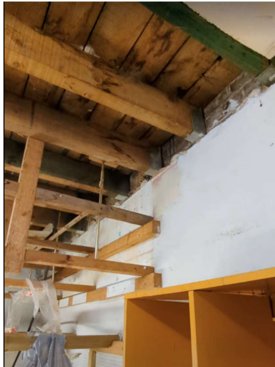
Image 15- Photograph of rear 1 st floor rear roof terrace from inside of the shop that is proposed to be replaced with new warm roof
