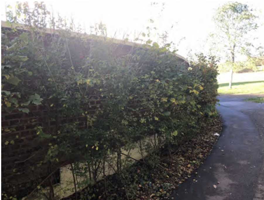
Figure 03 – View of the north eastern elevation of the boundary wall.
