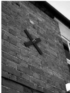
Figure 8: Traditional method restraint applied to bowing walls
