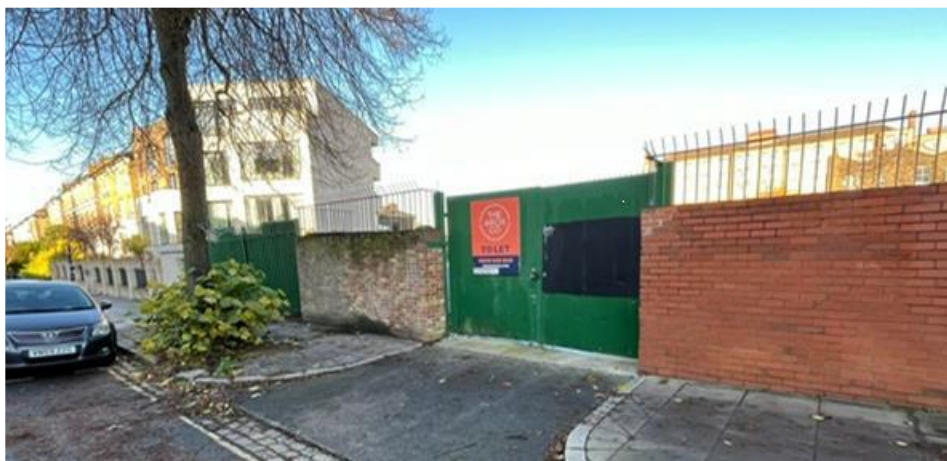
Frontage to the site showing access
