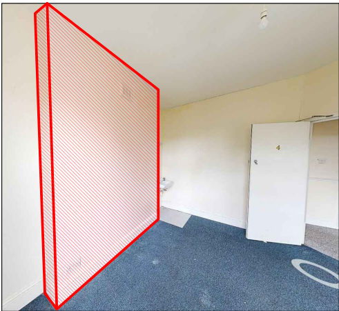
PARTITION DEMOLITION ON BEDROOM 05 & REMOVAL OF EXISTING SINK
