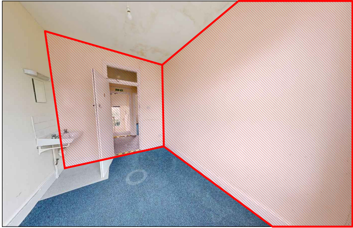
PARTITION DEMOLITION ON BEDROOM 06 & REMOVAL OF EXISTING SINK
