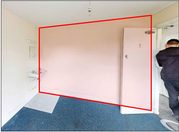
PARTITION DEMOLITION ON BEDROOM 07 & REMOVAL OF EXISTING SINK
