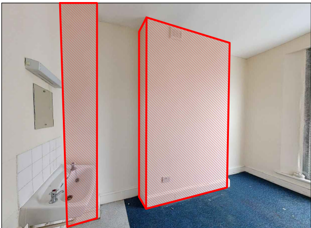
PARTITION DEMOLITION ON BEDROOM 04 & REMOVAL OF EXISTING SINK
