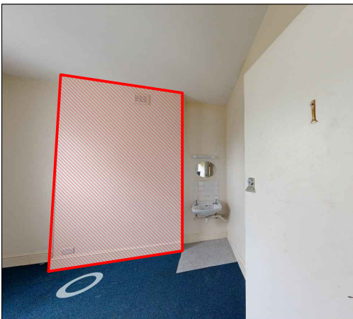
PARTITION DEMOLITION ON BEDROOM 03 & REMOVAL OF EXISTING SINK
