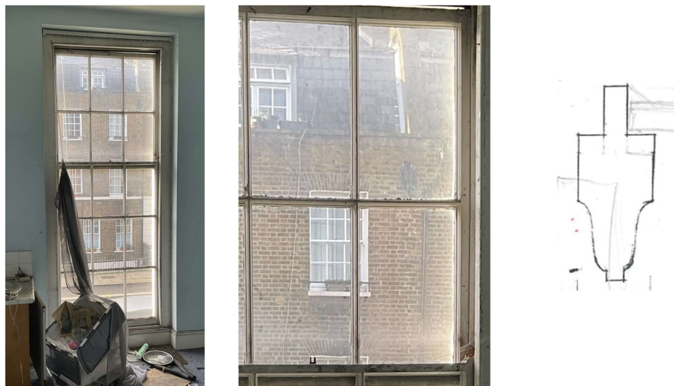
Pre-existing single glazed sashes and detail of the glazing bar and joinery profile to be reinstated
