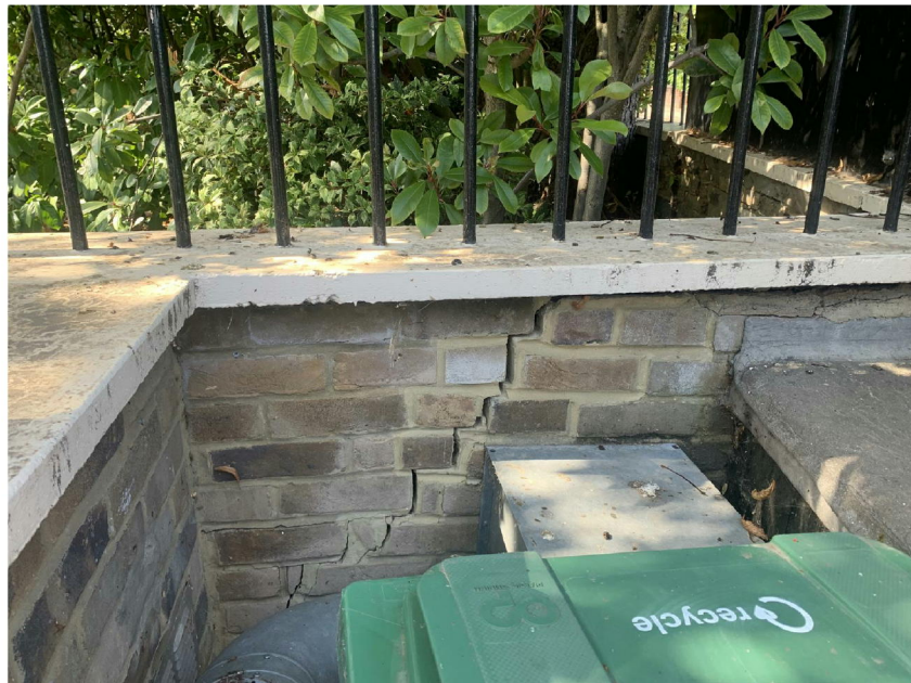
Cracking to perpendicular wall near Drive end
