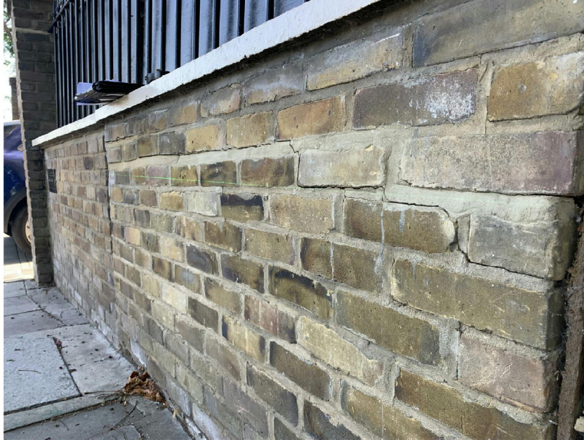
Panel H – Cracking, bulging out and tilt down to left (as shown by laser line)
