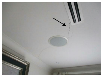
Cracking to ceiling in rear left hand bedroom
