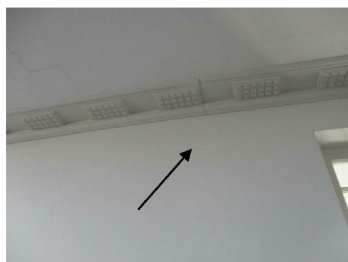
Cracking in hallway
