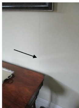
Cracking to dining room partition in sitting room
