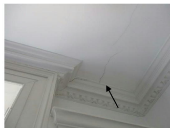
Cracking to ceiling / coving in ground floor study
