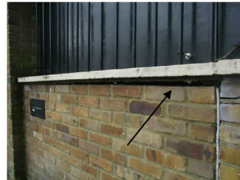
View of movement to front boundary wall
