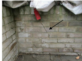
Cracking to garden retaining wall
