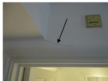
Cracking above en-suite door in rear left hand bedroom
