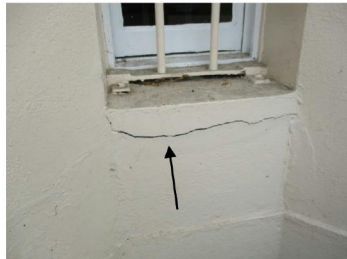
Cracking to rear kitchen bay
