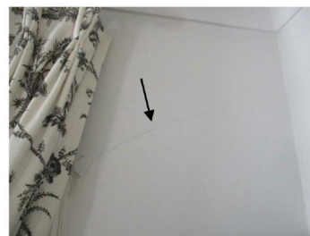
Cracking to rear wall in rear left hand bedroom
