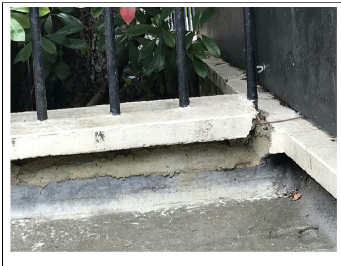
View of crack displacement
