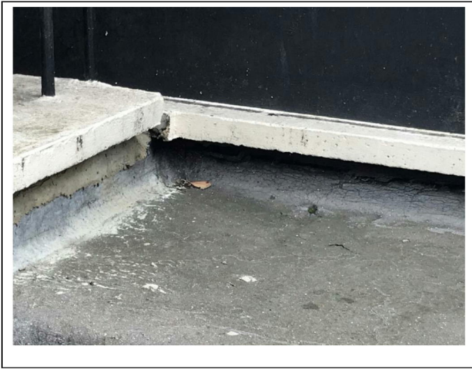
View of crack displacement
