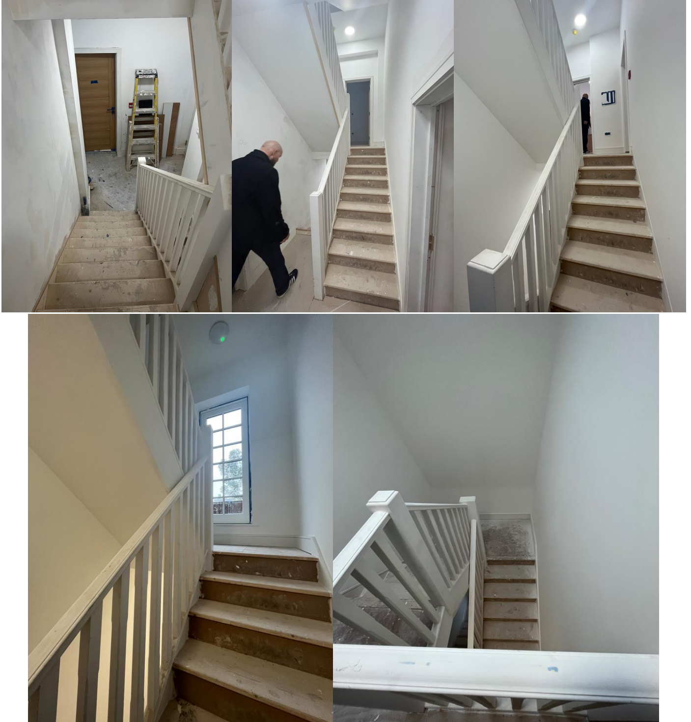
Replacement staircases – basement to third floor levels.
