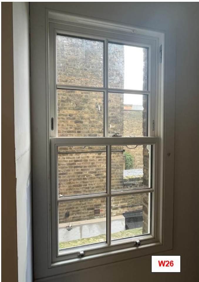
No.18 [left] & 20 [right]: TWO unauthorised laminated timber/composite sash windows ( W26 & W27 ) - first floor.
