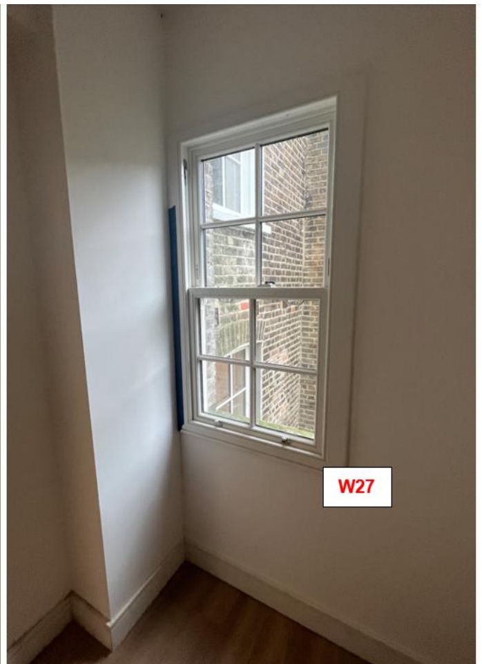
No.18 [left] & 20 [right]: TWO unauthorised laminated timber/composite sash windows ( W26 & W27 ) - first floor.
