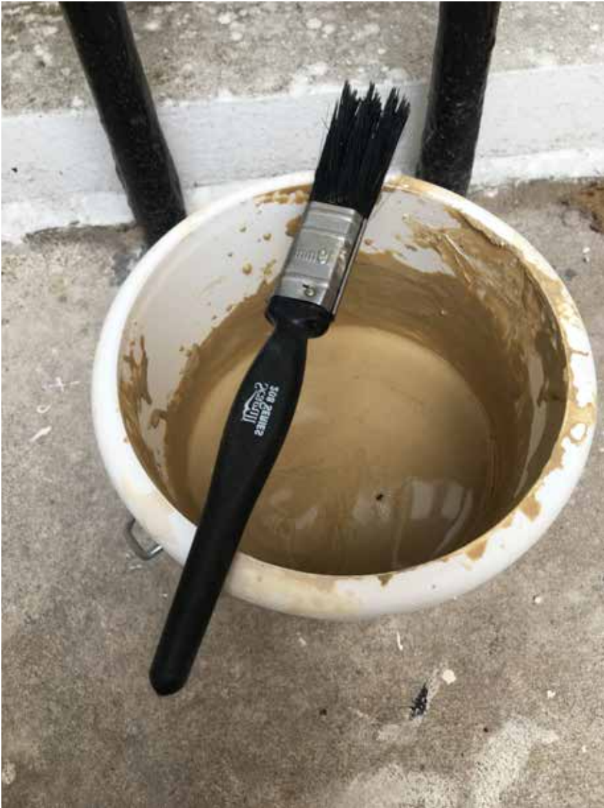
A 19mm brush was generally used for tinting the repairs.
