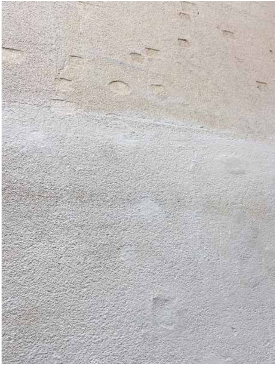
The repair mortar has been rubbed down and limewash applied to the extent of the stone joints. The repair is not yet satisfactory.
