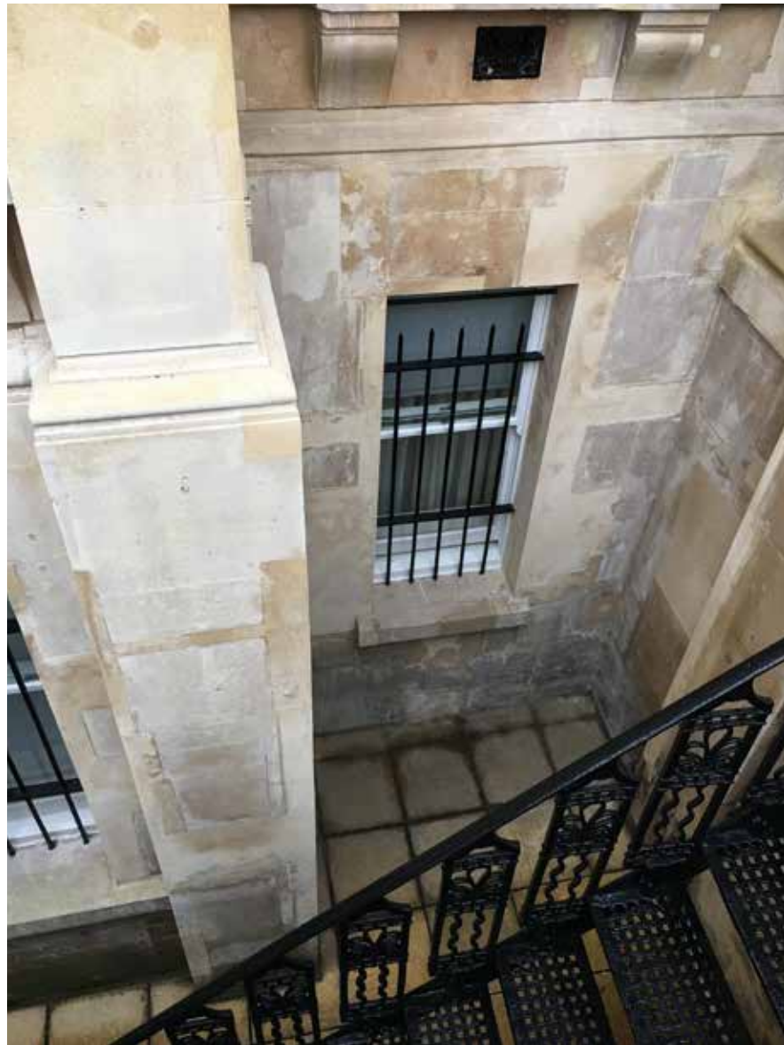
Stone in basement areas frequently displays extensive variability in colour.
