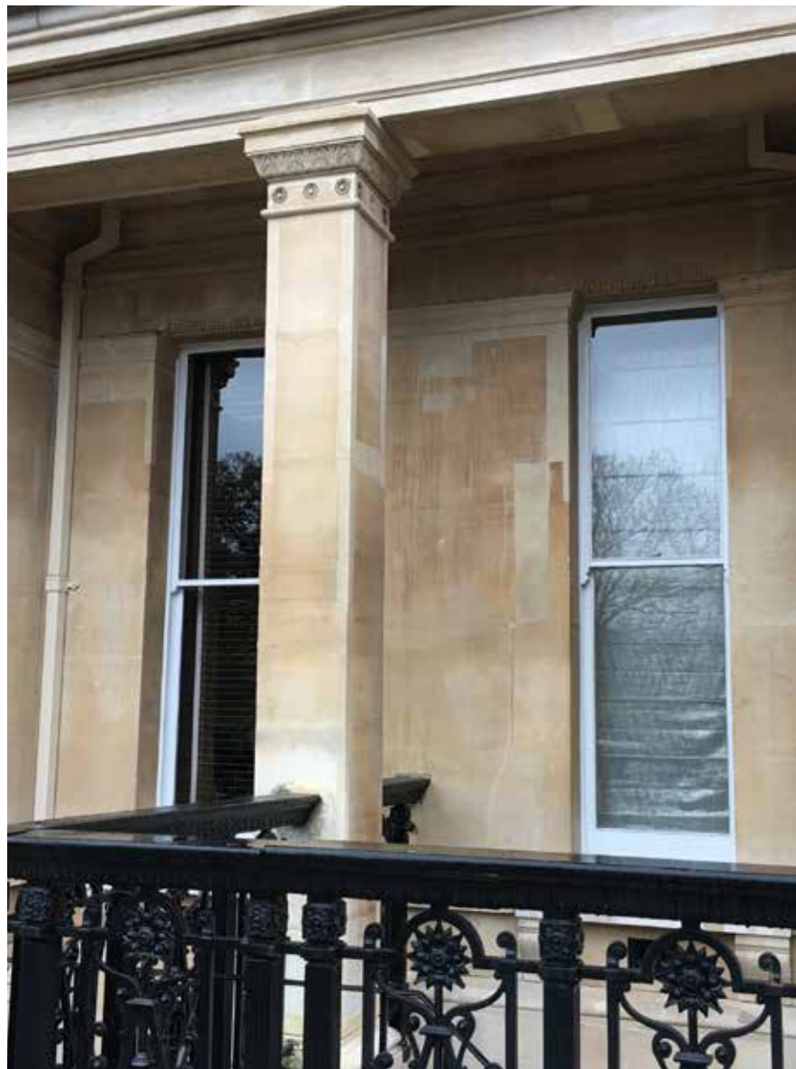
Large mis-matched mortar repairs in recessed bays.
