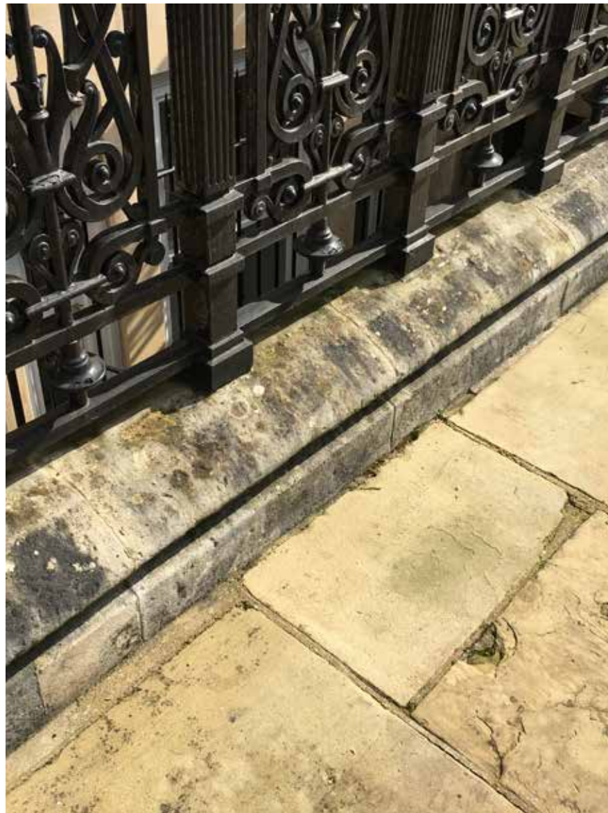
The heavily soiled stone plinths below the railings is to be cleaned.
