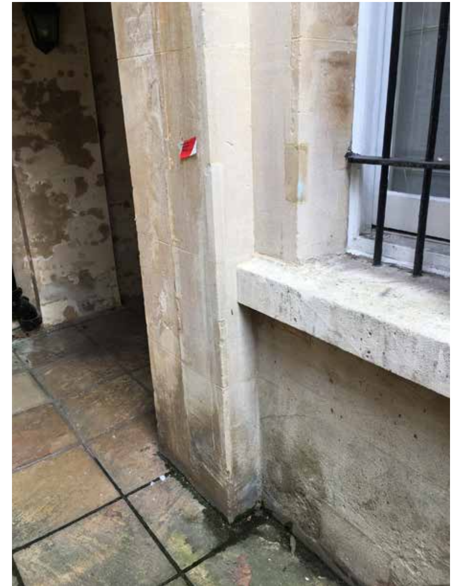
View from three metres. The dark colour of the pre-existing repair can be seen in the untreated corner repair to the right.
