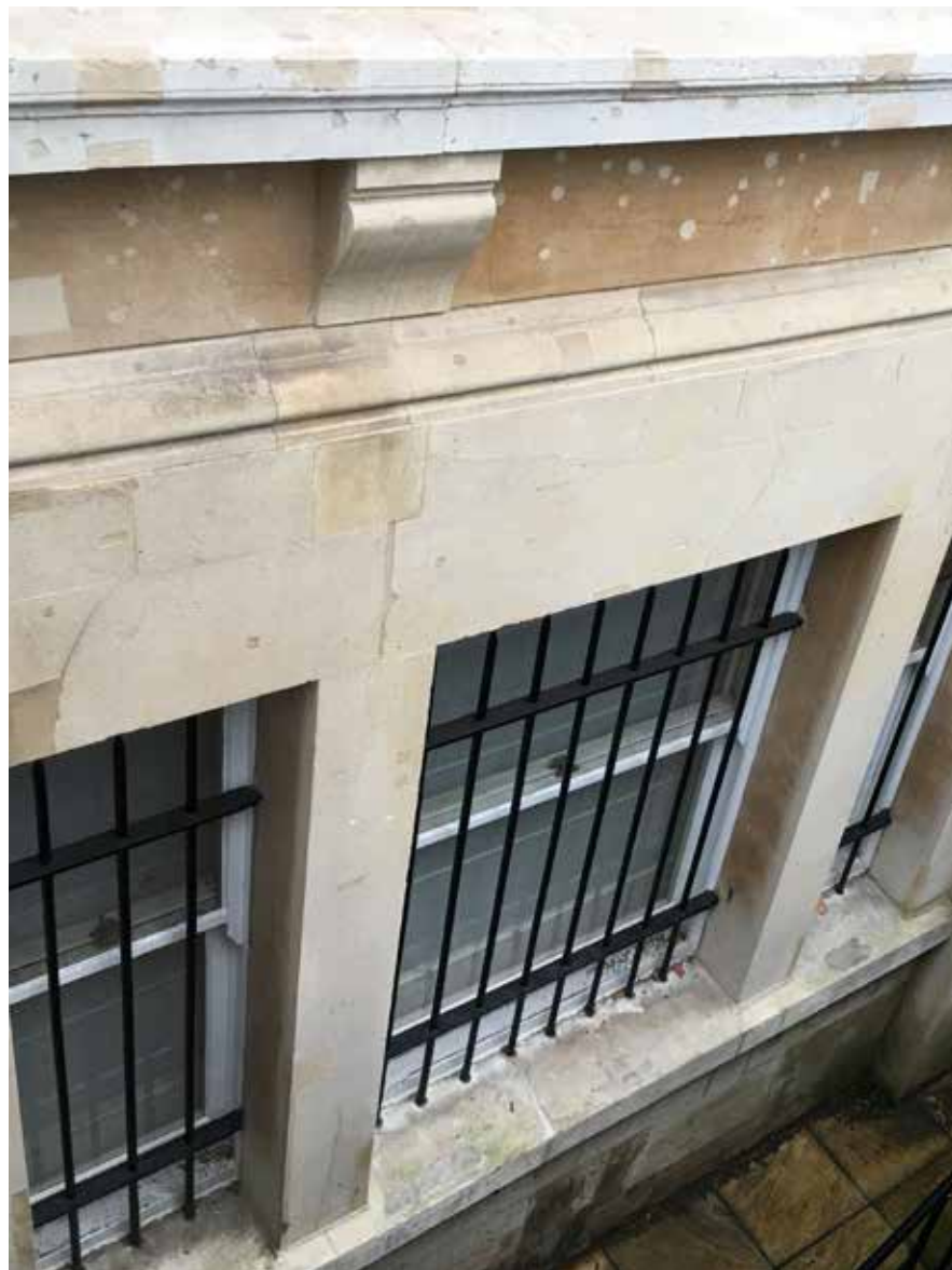
Pre-existing contrasting repairs under the window sill of House 5.
