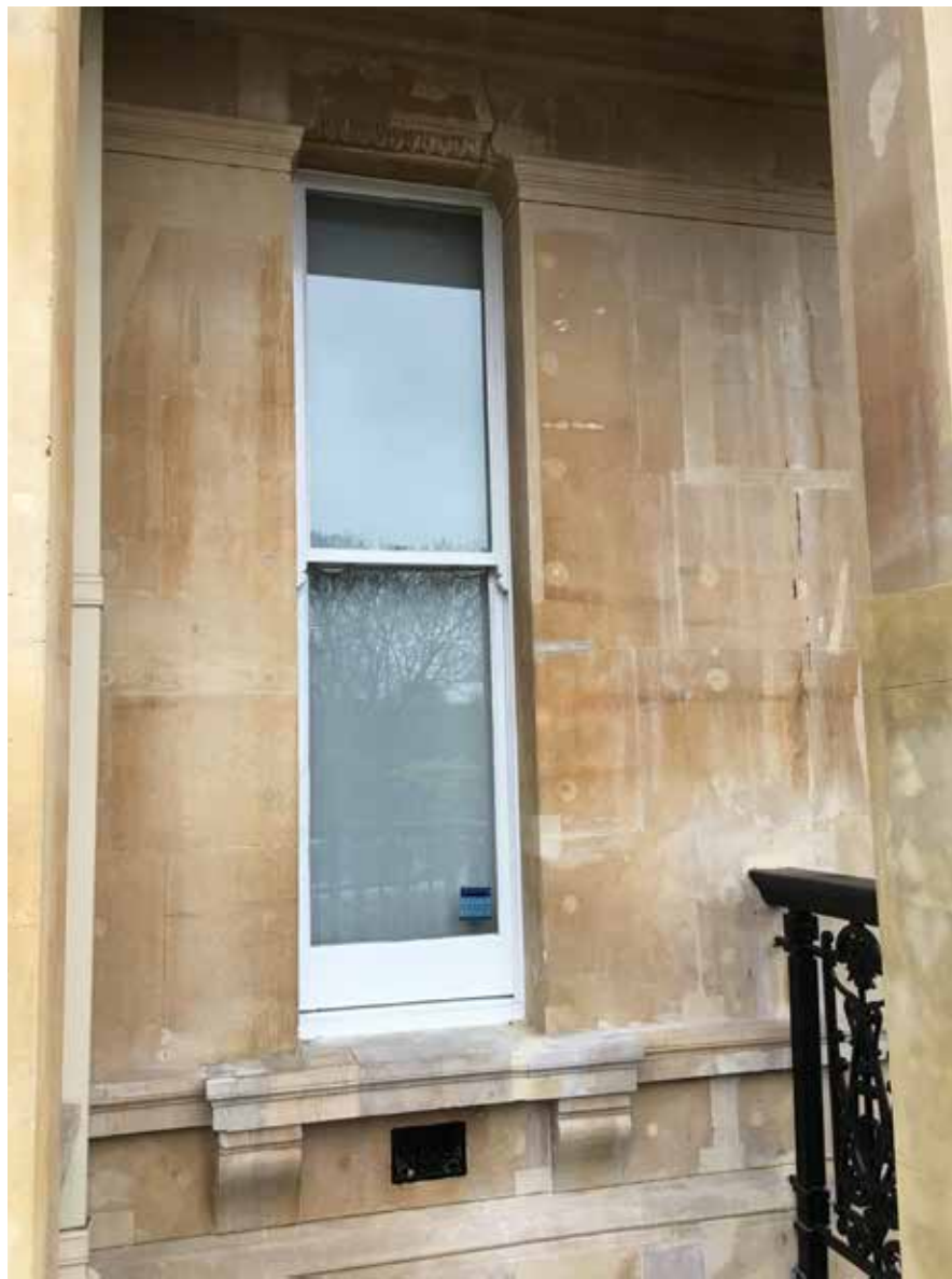
Pockmarked appearance of mortar repairs in recessed bays.
