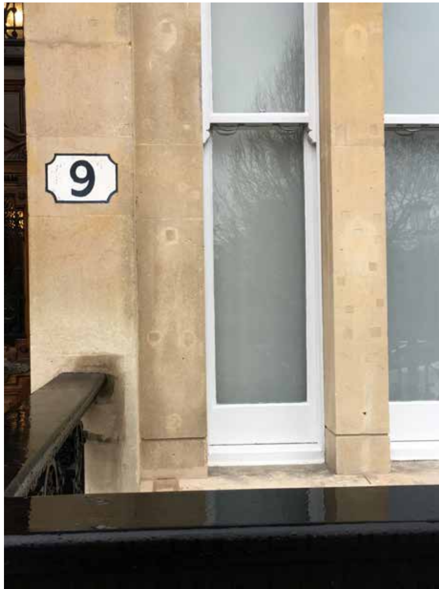
In this instance the repairs are a good match to the underlying stone, but rubbing down the repair has lightened the surrounding stone to give a 'hallow' effect.
