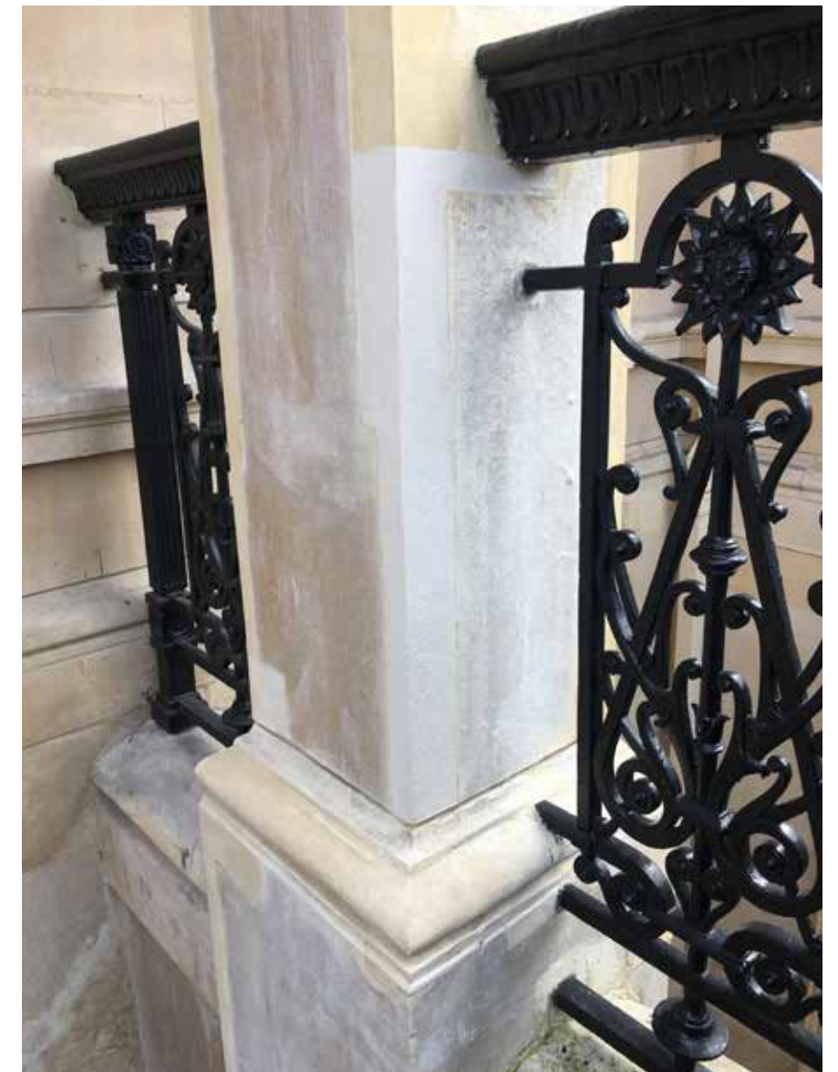
The corner repair after ten days. The side facing outwards is considered satisfactory, while the lateral face still has a strong contrast to the darker adjacent stone.
