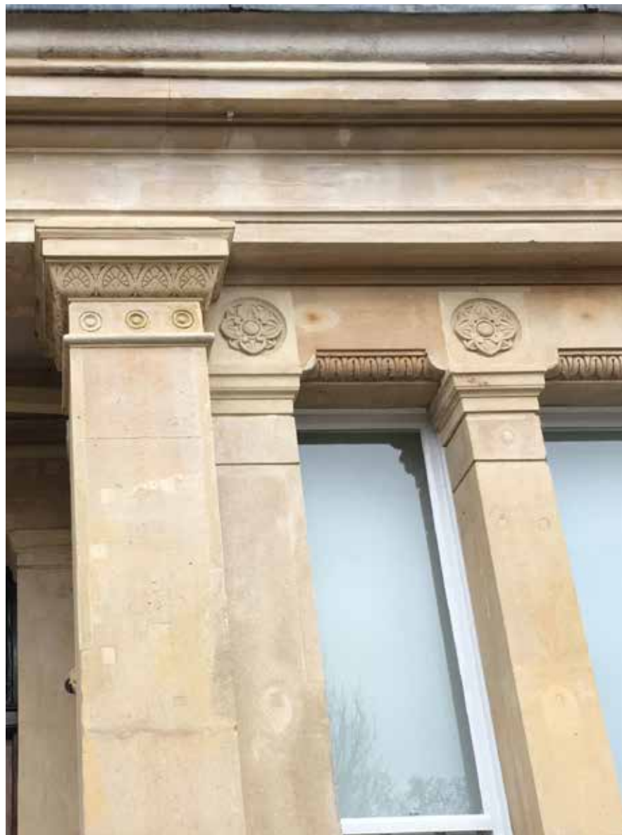
High-level poorly-matched repairs of moulded rosettes.
