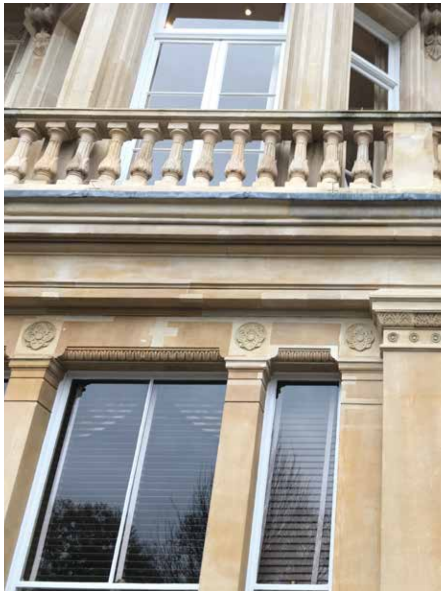
High-level poorly-matched repairs of moulded rosettes.
