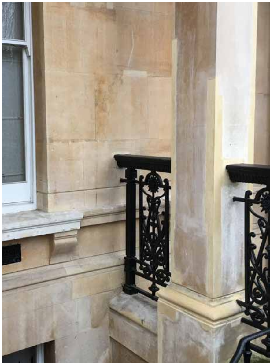
Poor colour match of corner repairs to pillar.
