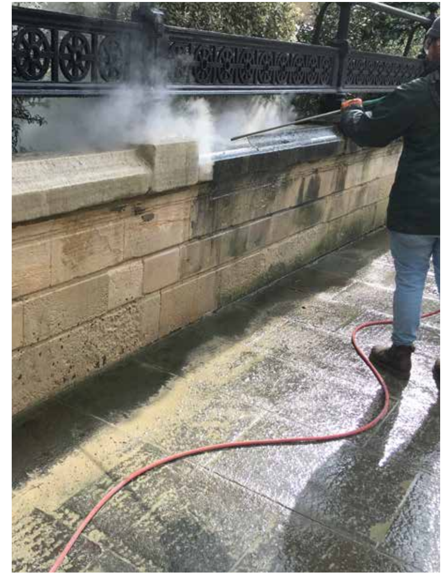
The Bath stone perimeter wall to the Outer Circle has recently been cleaned by Doff steam cleaning.
