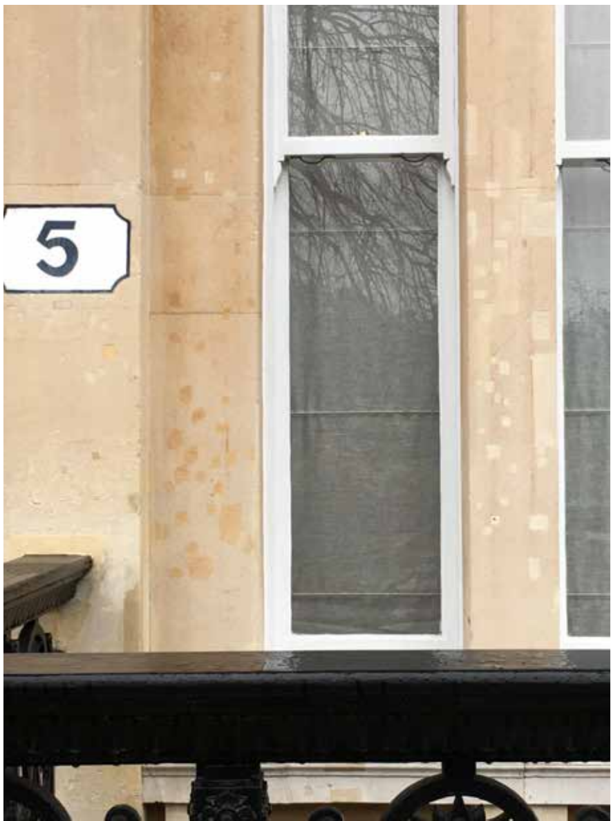
Small-scale repairs do not match the dark or lighter stone.
