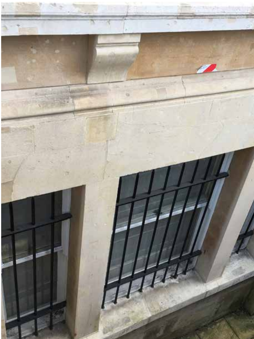
The remediated tinted repairs under the window sill of House 5. The area to the right of the bracket has been treated, while the area to the left of the bracket is untouched. These repairs are considered satisfactory.
