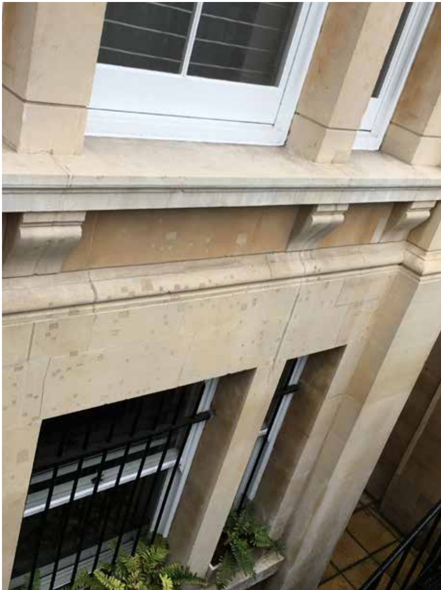
The repair mortar on the dark stone is too light and the repair mortar on the light stone is too dark.
