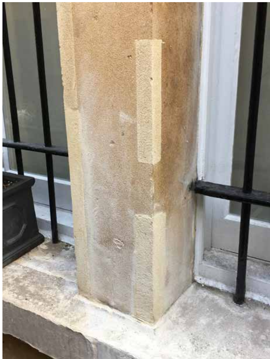
The pre-existing contrasting corner repair in the basement area of House 5 is very much lighter than the surrounding dark stone.
