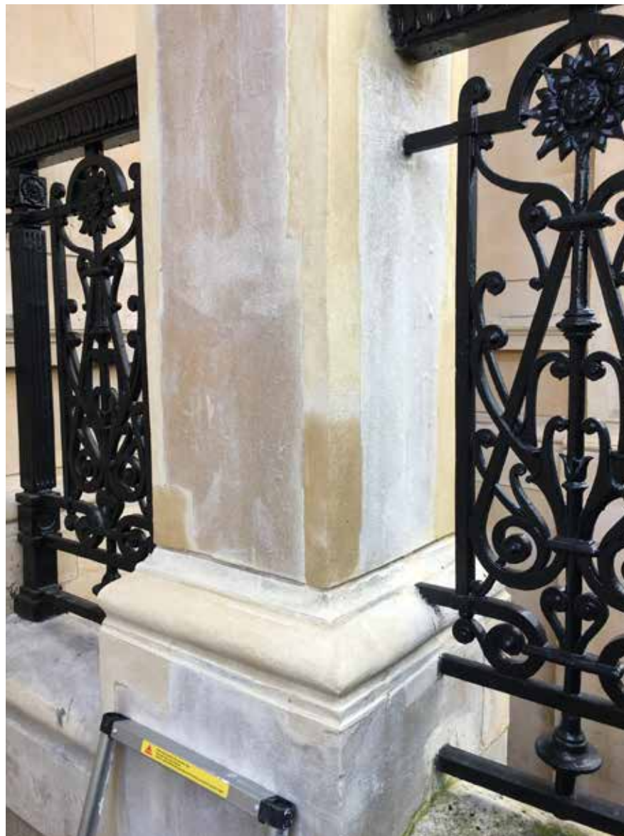
The pre-existing contrasting corner repair at the column base between House 5 and House 6 has an orange tinge. The outward face of the column has weathered to a very light colour, while the side of the column remains dark.
