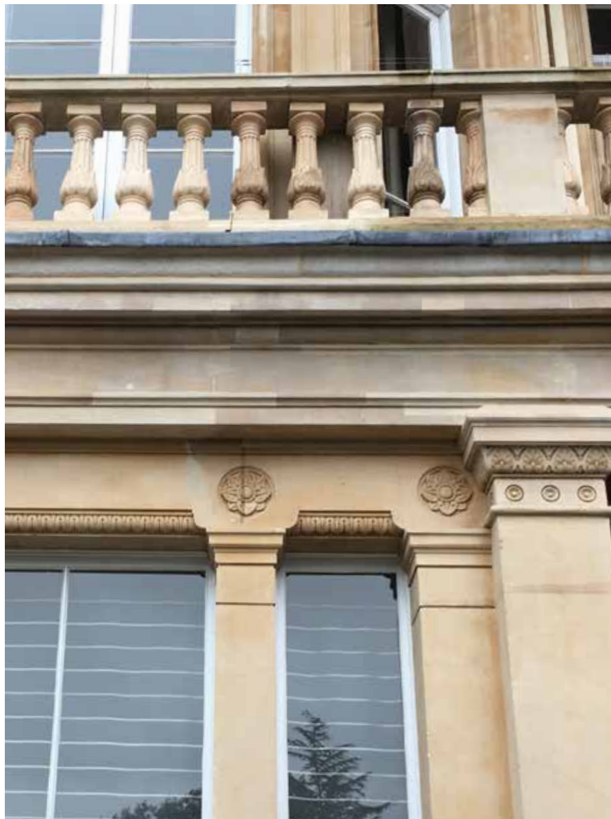
High-level poorly-matched repairs of cornice.
