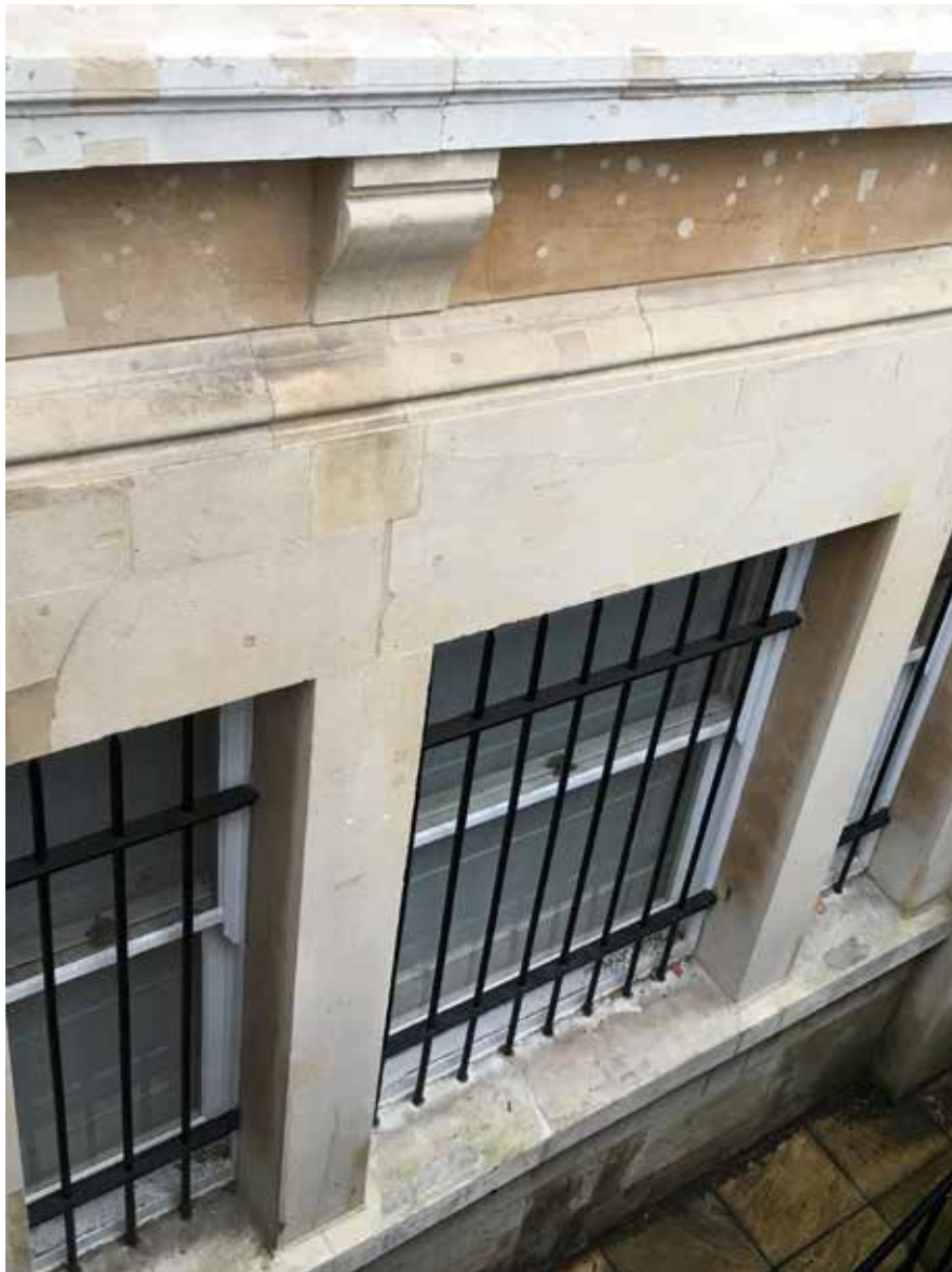
In this case the repair mortar on the dark stone is also too light.
