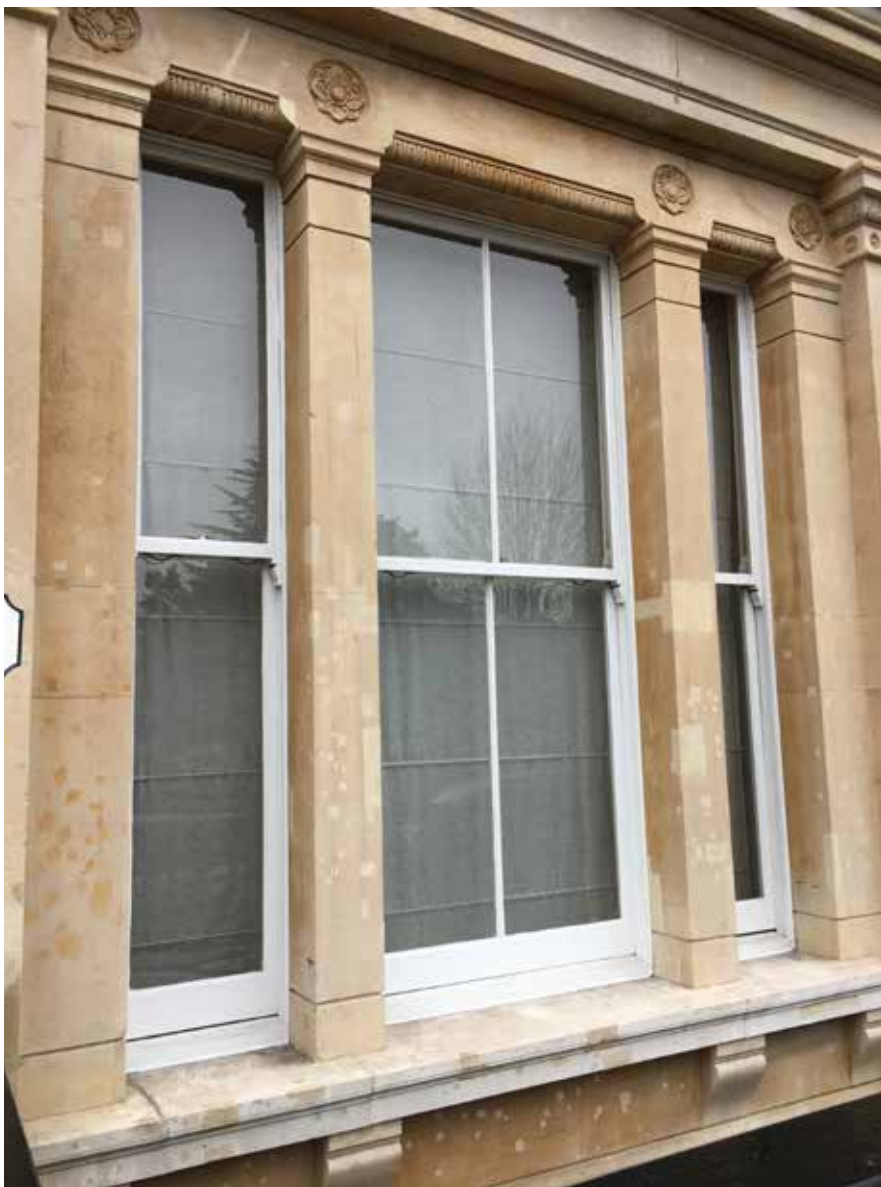
Many small poorly-matched pockmark repairs across a window bay.
