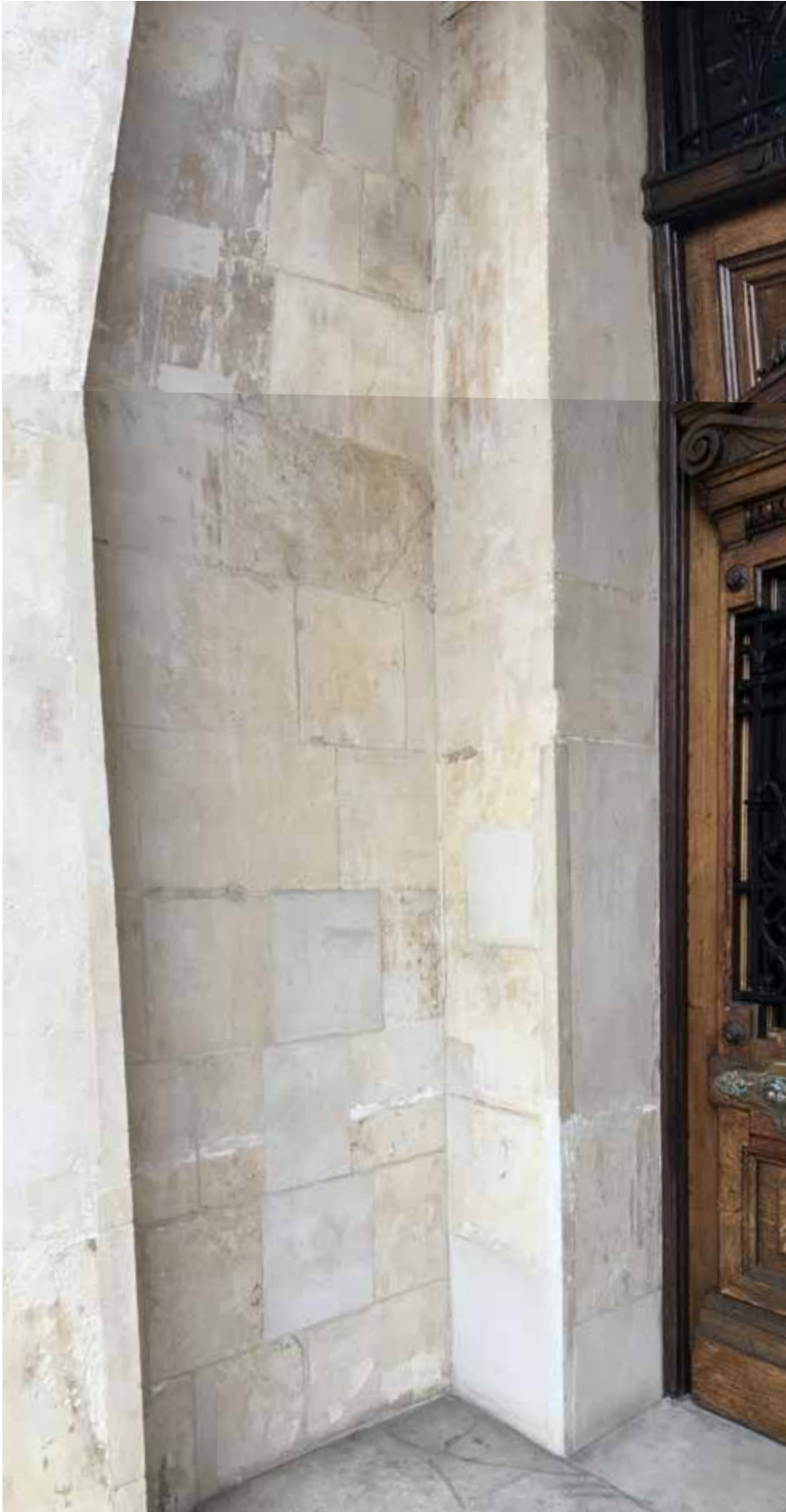
Extensive repairs and poor surface finish to the recessed entrance .
