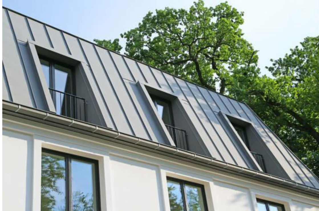
Zink Patina standing seam to mansard elevations.
