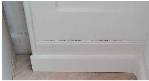
Photograph of existing "Type 4" skirting boards
