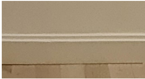
Photograph of existing 'Type 3' skirting boards
