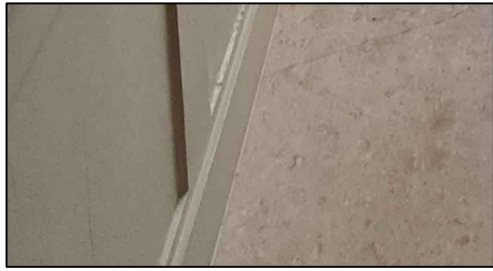
Photograph of existing 'Type 6' detail to shower room
