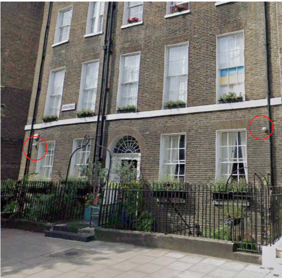
Two dome CCTV cameras installed to the front facade of No. 28 John Street which is within the same group listing as No. 22 John Street.
