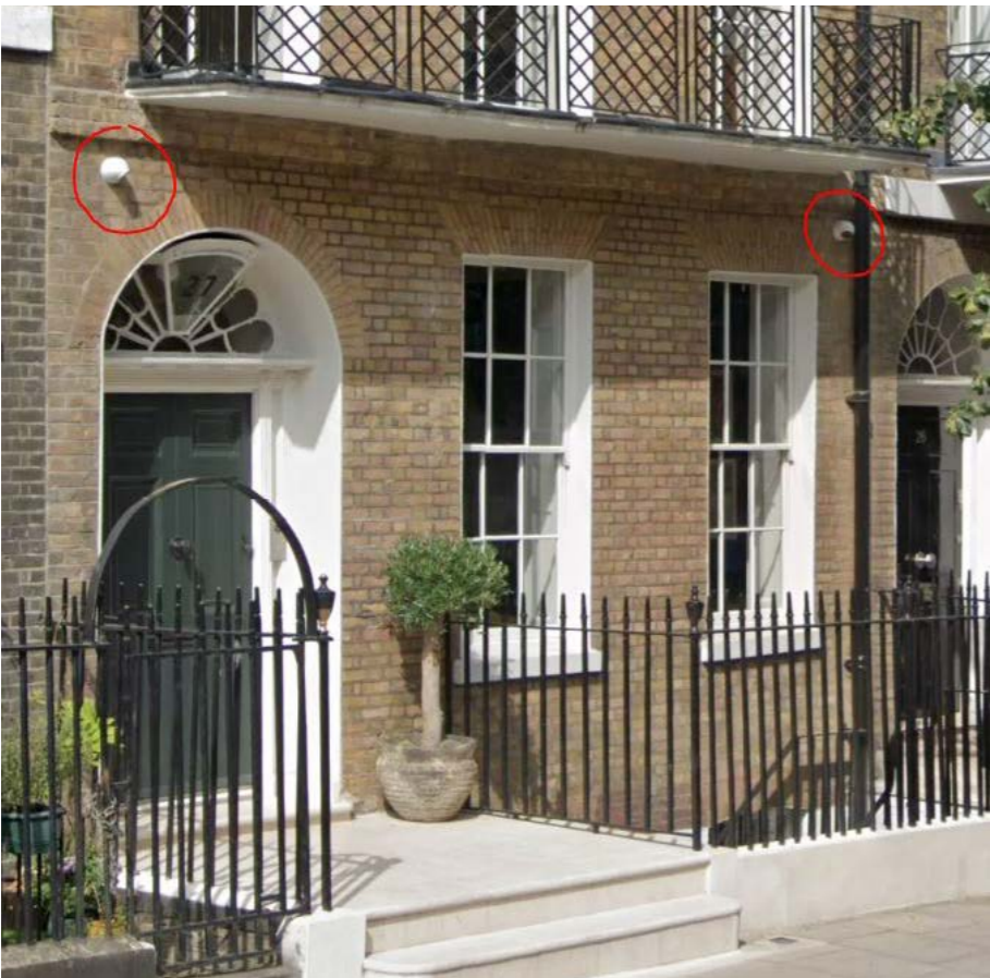
Two dome CCTV cameras installed to the front facade of No. 27 John Street which is within the same group listing as No. 22 John Street.
